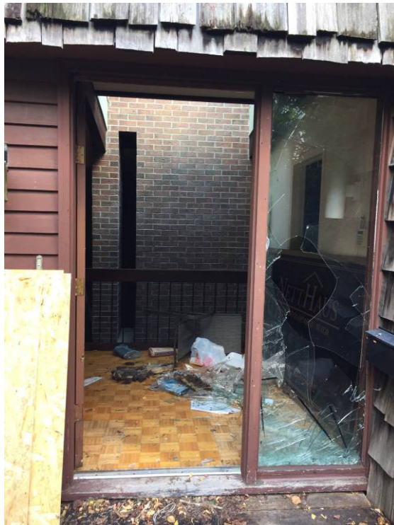
Figure 12. Plywood removed, showing broken glass.
