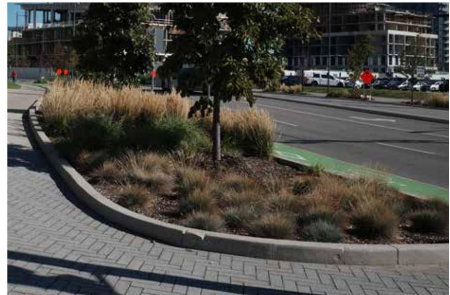
Fig. 119. Raised planter edges help protect street trees from salt splash.
