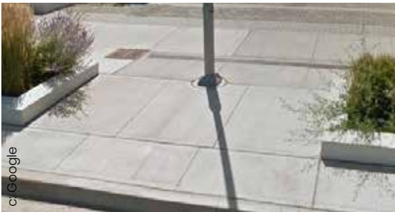
Fig. 123. Poured in place concrete with sawcut jointing.
