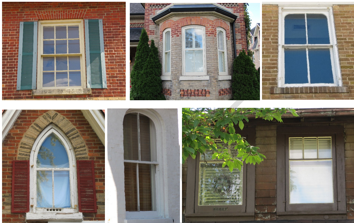
Photo 4.5: Original window examples in HCD including rectangular multi-sash, segmental storm windows, semi-elliptical sash, pointed arched, semi-circular sash, and rectangular 3/1
