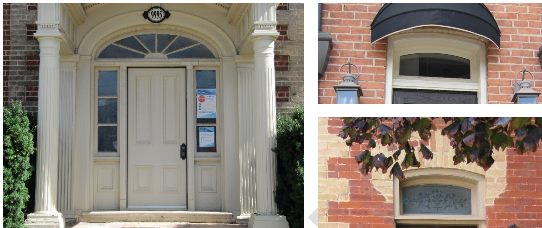
Photo 4.6: Examples in HCD of original door sidelights, fanlight, mouldings, and segmental transoms
