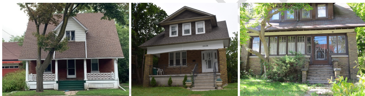
Photo 4.8: Examples of covered wood full-width front porches on Keele Street north of Major Mackenzie Drive West
