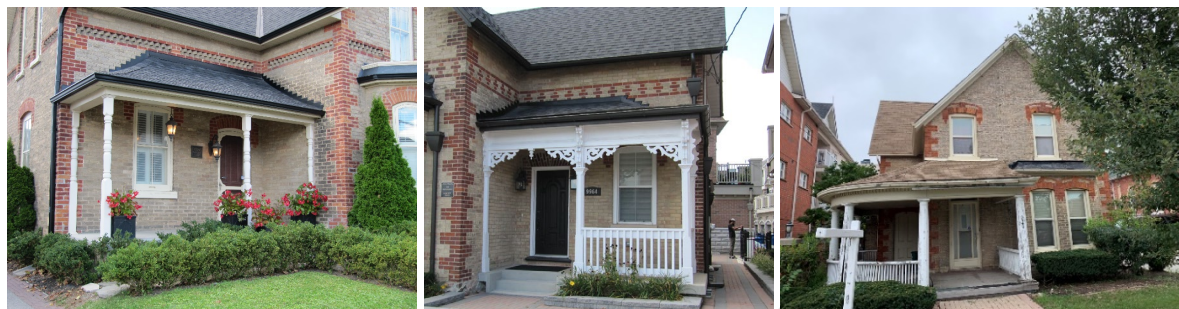
Photo 4.7: Examples of covered partial wood front porches on Keele Street south of Major Mackenzie Drive West
