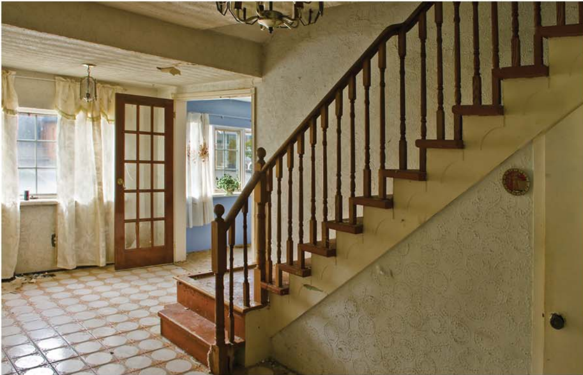
Entry Hall Looking North - West: Showing The Incorporated Enclosed Front Porch Indicated By The Drop In The Ceiling, The Newer Stairs In The Original Location, And No Original Trim
