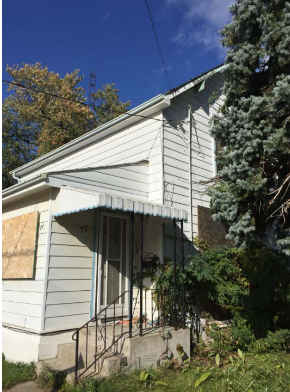
Front Entrance of 77 Clarence Street
