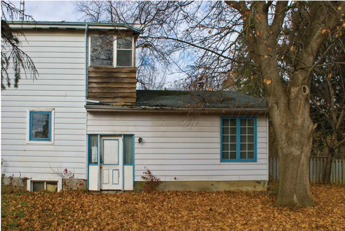
South Elevation Of The Kitchen Section Of The Two - Floor House, And The Rear Addition: Showing The Side Entry Door With Side Lights, And The Enclosed Deck Off The Second Floor Master Bedroom
