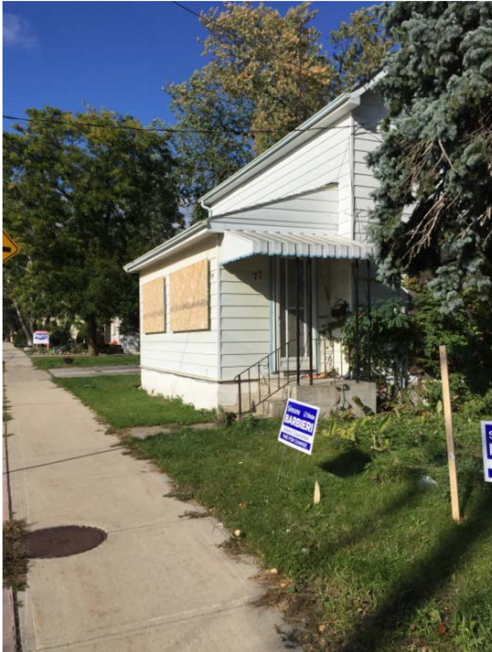
Front view of 77 Clarence Street
