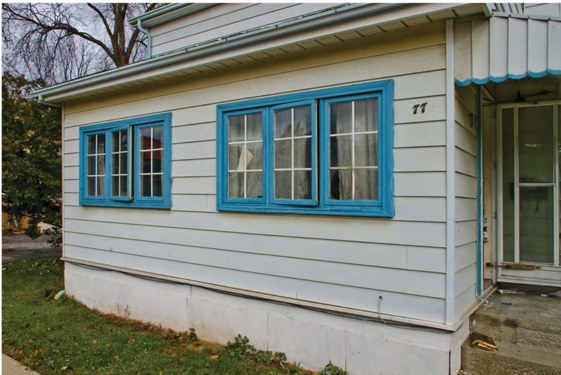
West Elevation Of The Enclosed Front Porch, And A Portion Of The New Front Entry
