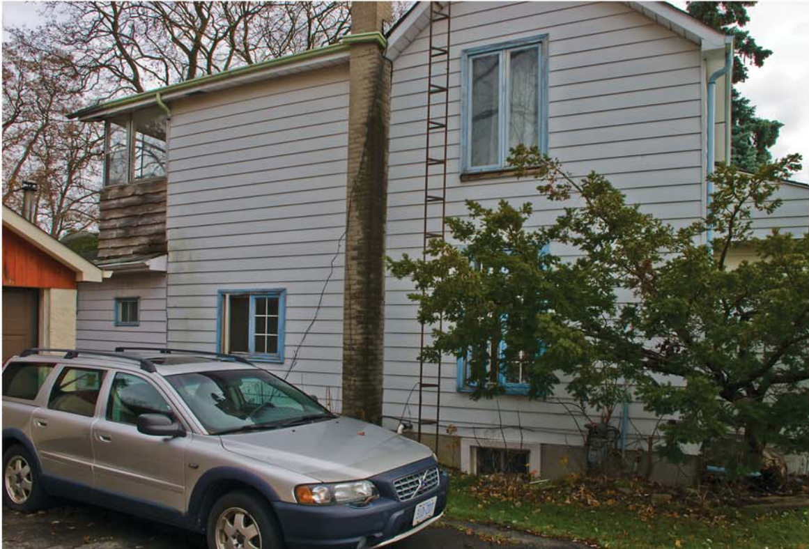
North Elevation Showing Metal Siding, Soffits & Fascia, Enlarged Window On The Second Floor, & Brick Chimney
