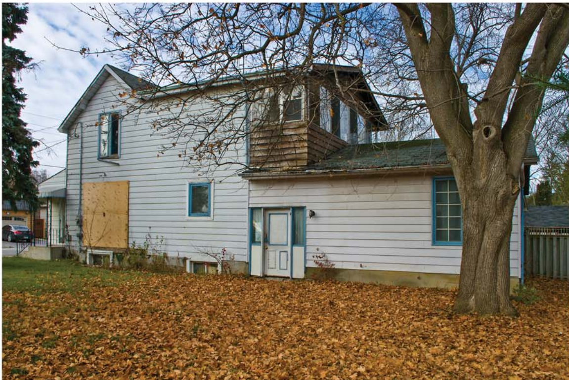
Original Two - Storey House Left, Kitchen Section Middle, And Newer Addition Right
