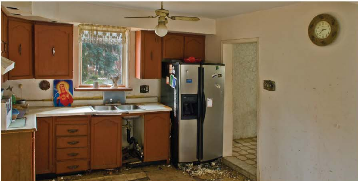
Kitchen Looking South - West: Step Up To The Front Entry Can Be Seen On The Right
