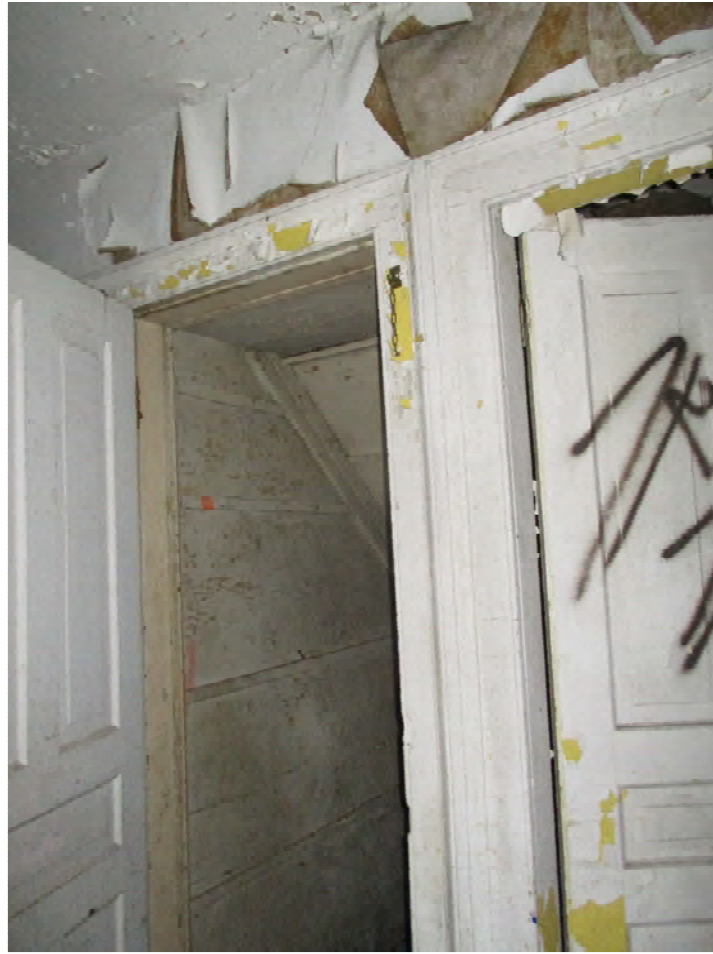
Casing and backband on a pair of doors
