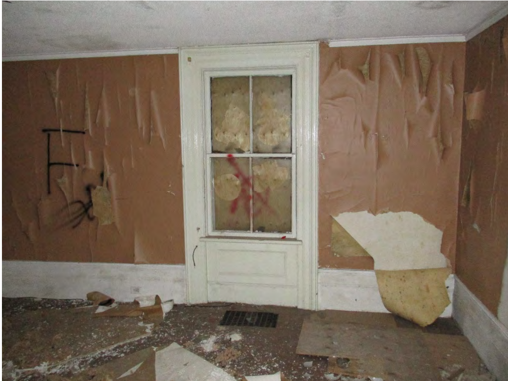
Casing, panel, and baseboard in north front room
