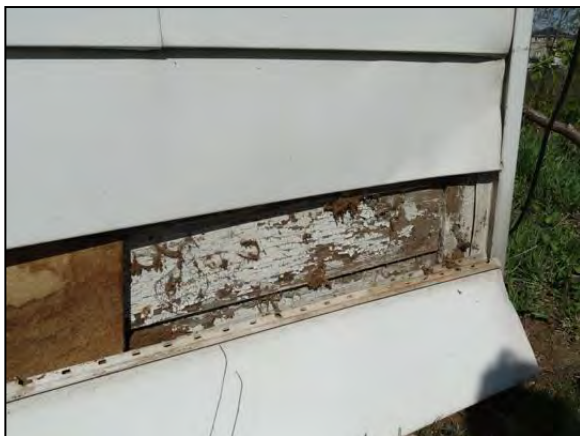
Figure 9: Exposed wood clapboard beneath metal cladding, 2016
