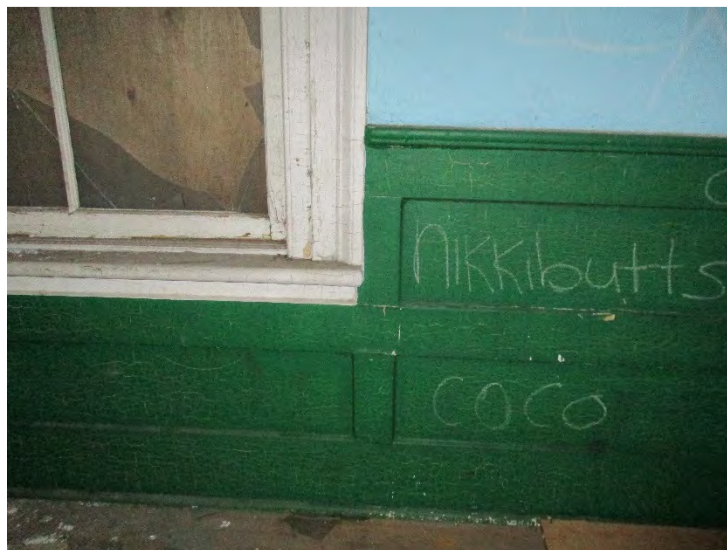
Later paneled wainscot butted to original window casing
