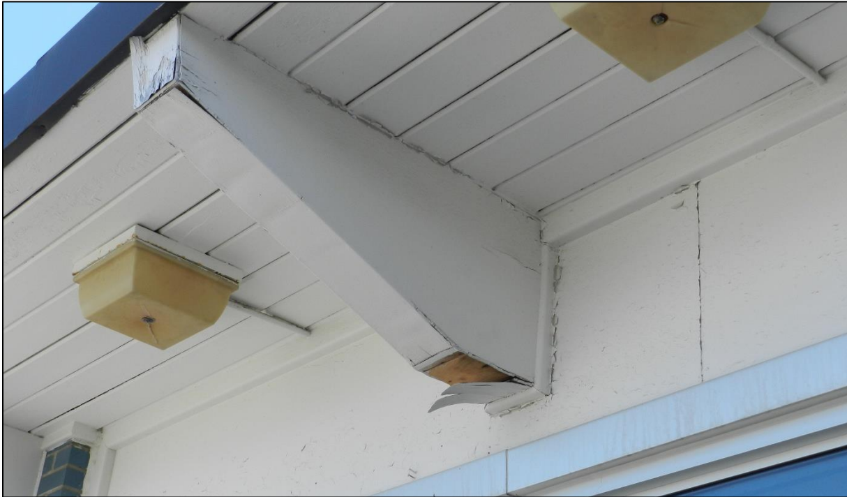
Figure 25: Detail of the roof overhang and wooden plank soffit supported by tapered wooden beams clad in plywood (ASI 2020)
