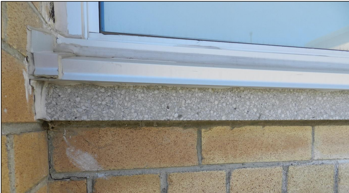
Figure 24: Detail of the precast concrete sills clad in metal (ASI 2020)
