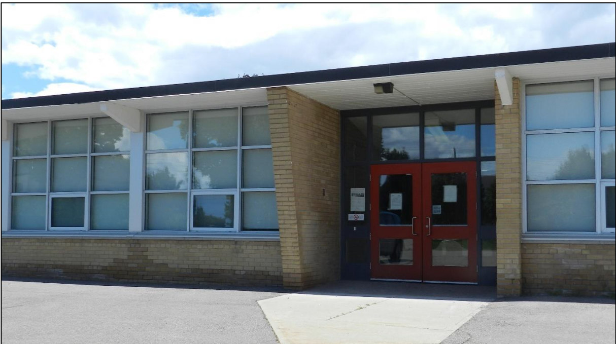
Figure 26: Recessed entrance with double-doors surrounded by a 3-pane transom window, and large side-lights, flanked by an articulated tapered brick on the south side, built of progressively corbelled bricks, and a brick pier on the north side. (ASI 2020)
