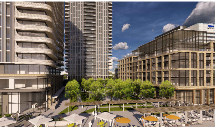
VIEW LOOKING EAST ACROSS COURTYARD
