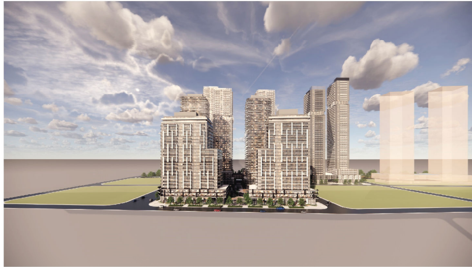
VIEW LOOKING WEST TOWARDS BUILDINGS 4 AND 5 FROM MAPLECRETE ROAD
