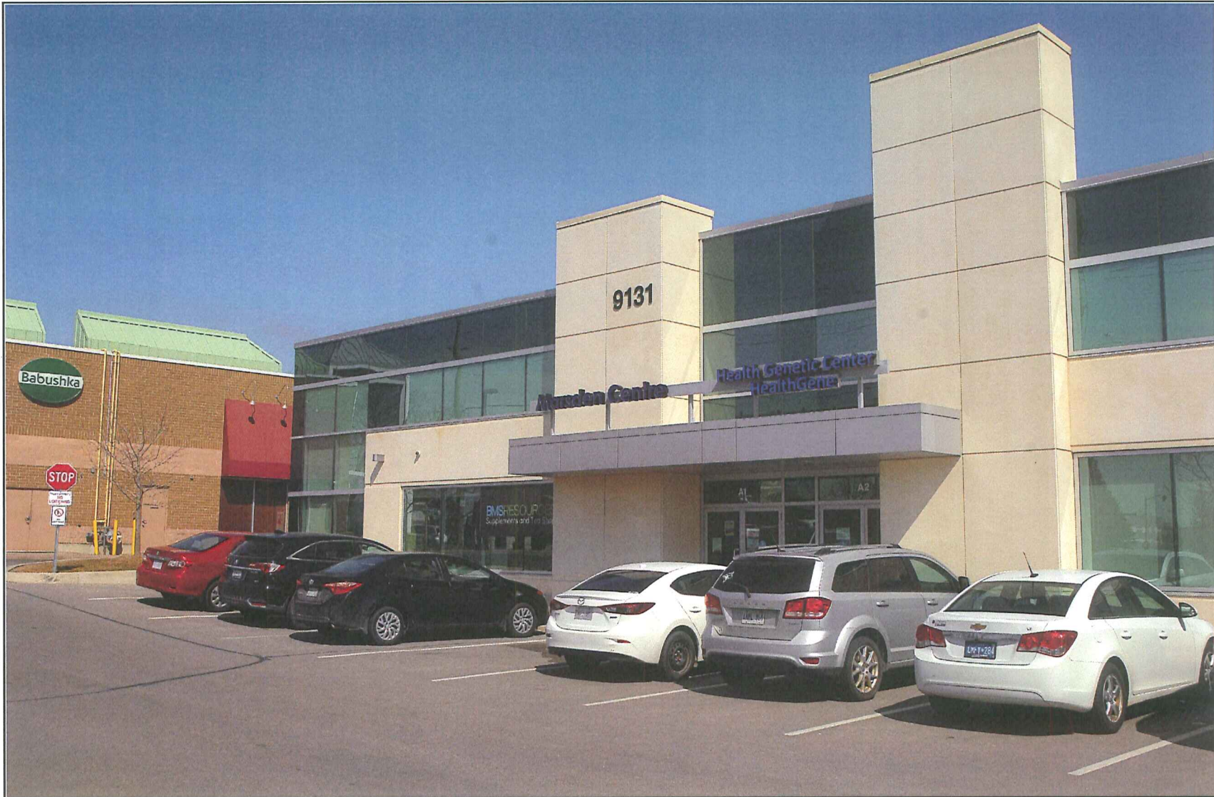
IMAGE 3: MARSDEN HEALTH CENTRE UNIT A1, FRONTING KEELE ST. 9131 KEELE ST. VAUGHAN
