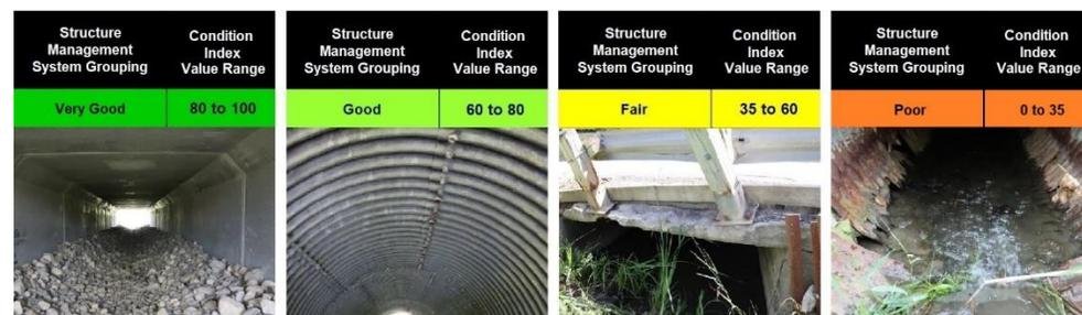
Figure 6-10: Images of Culvert Inspections Compared to Asset Management Condition Rating
