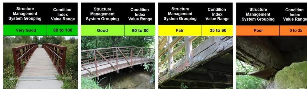
Figure 6-9: Images of Bridge Inspections Compared to Asset Management Condition Rating
