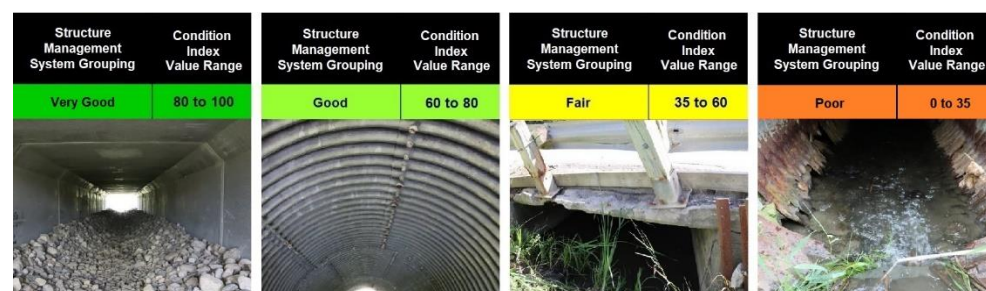
Figure 6-10: Images of Culvert Inspections Compared to Asset Management Condition Rating
