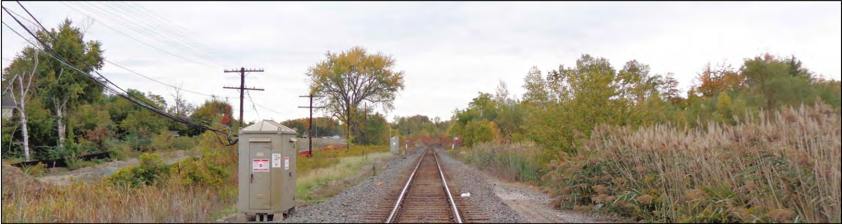
Canadian Pacific Railway right-of-way to the rear of the subject site; view looking southeast from near Nashville Road.
