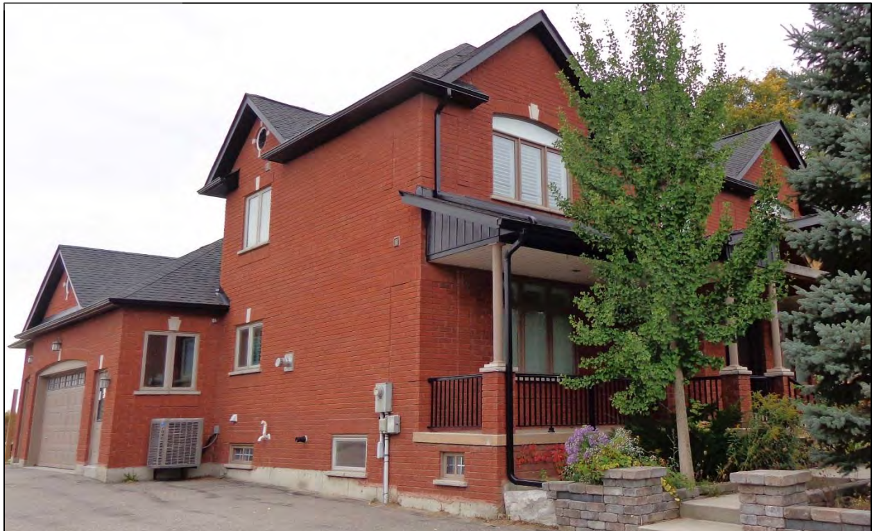
South and East Elevations
