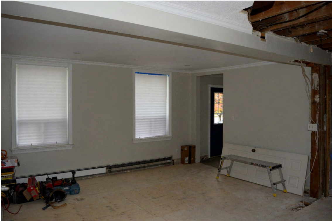
Image 14: First floor interior, note bulkhead indicating original location of internal wall, facing northwest
