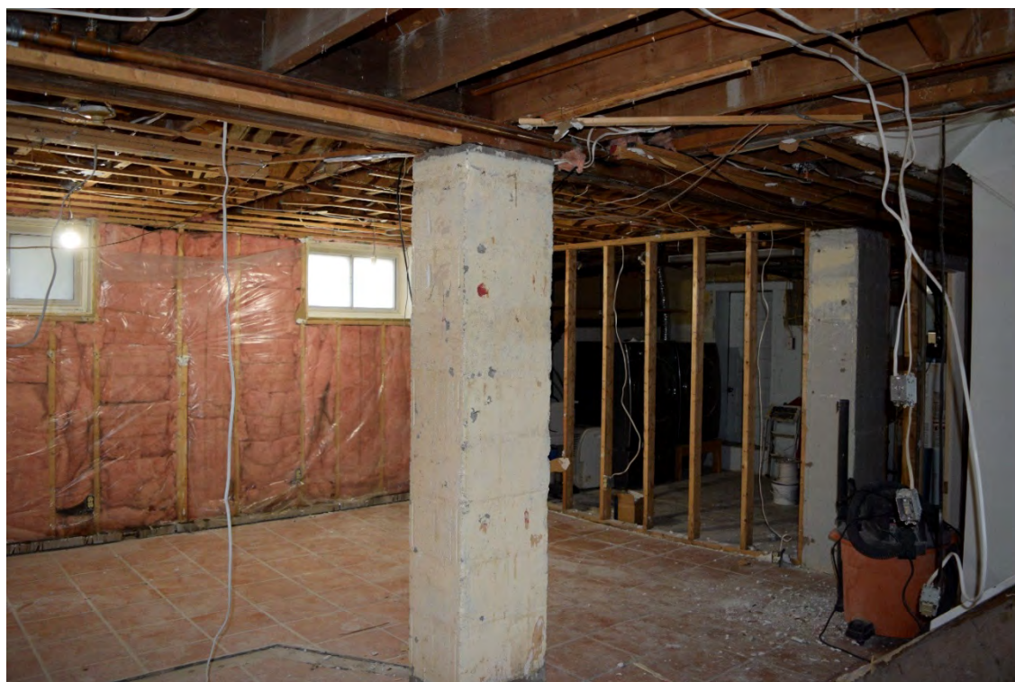
Image 23: Basement, note original cement block support pillars, facing northwest
