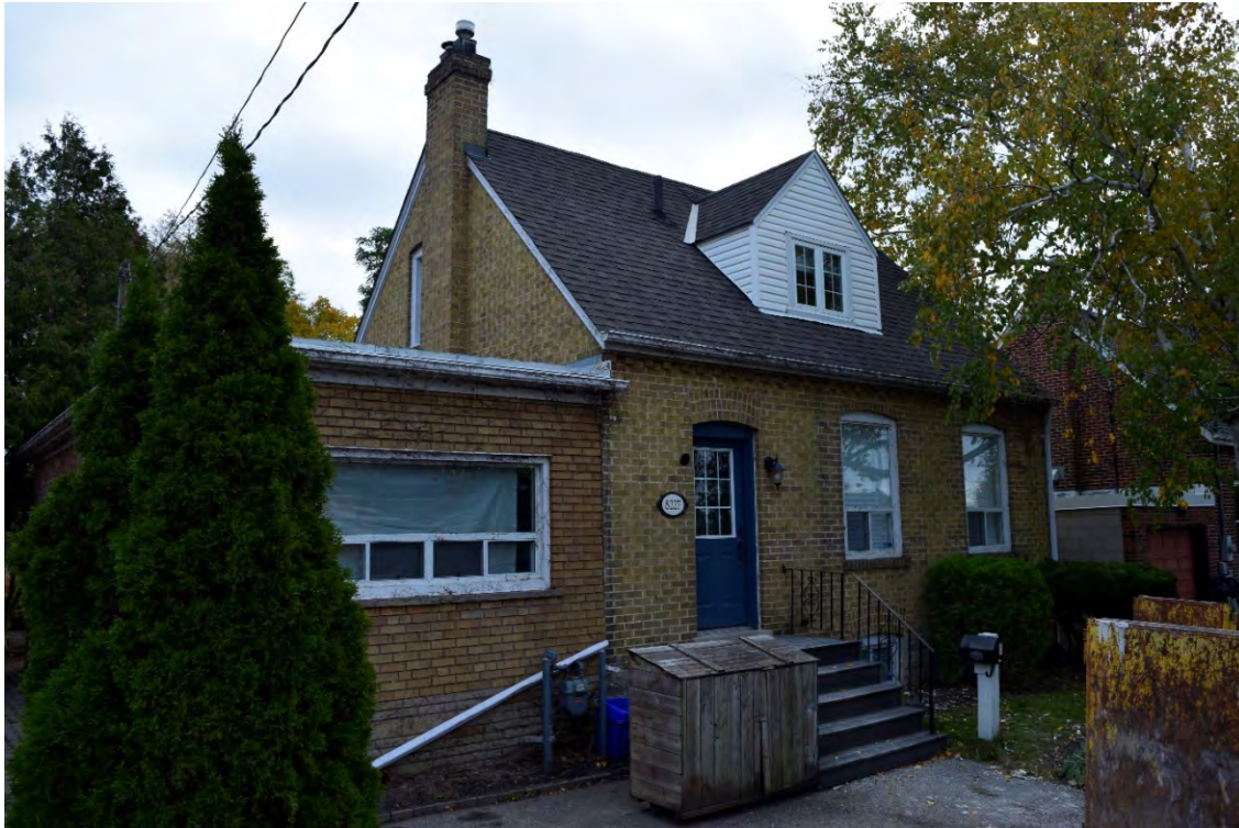
Image 3: Front façade of 8227 Kipling Avenue, facing east-southeast
