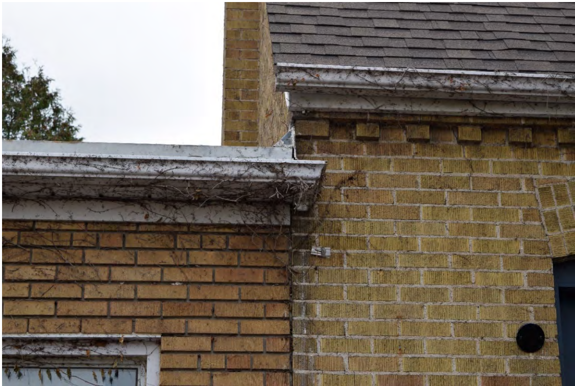
Image 7: Close up of seam occurring between north addition and original structure, note brick dentate at eave.
