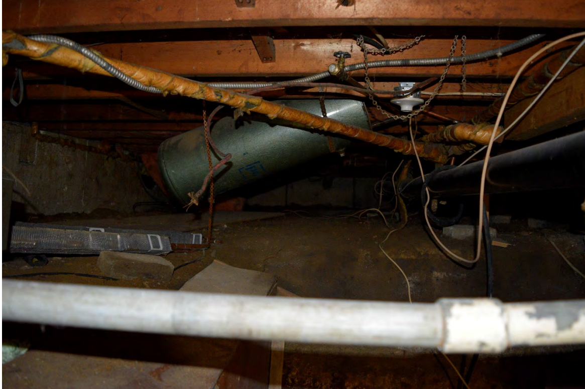
Image 25: Crawl space under north addition, facing west
