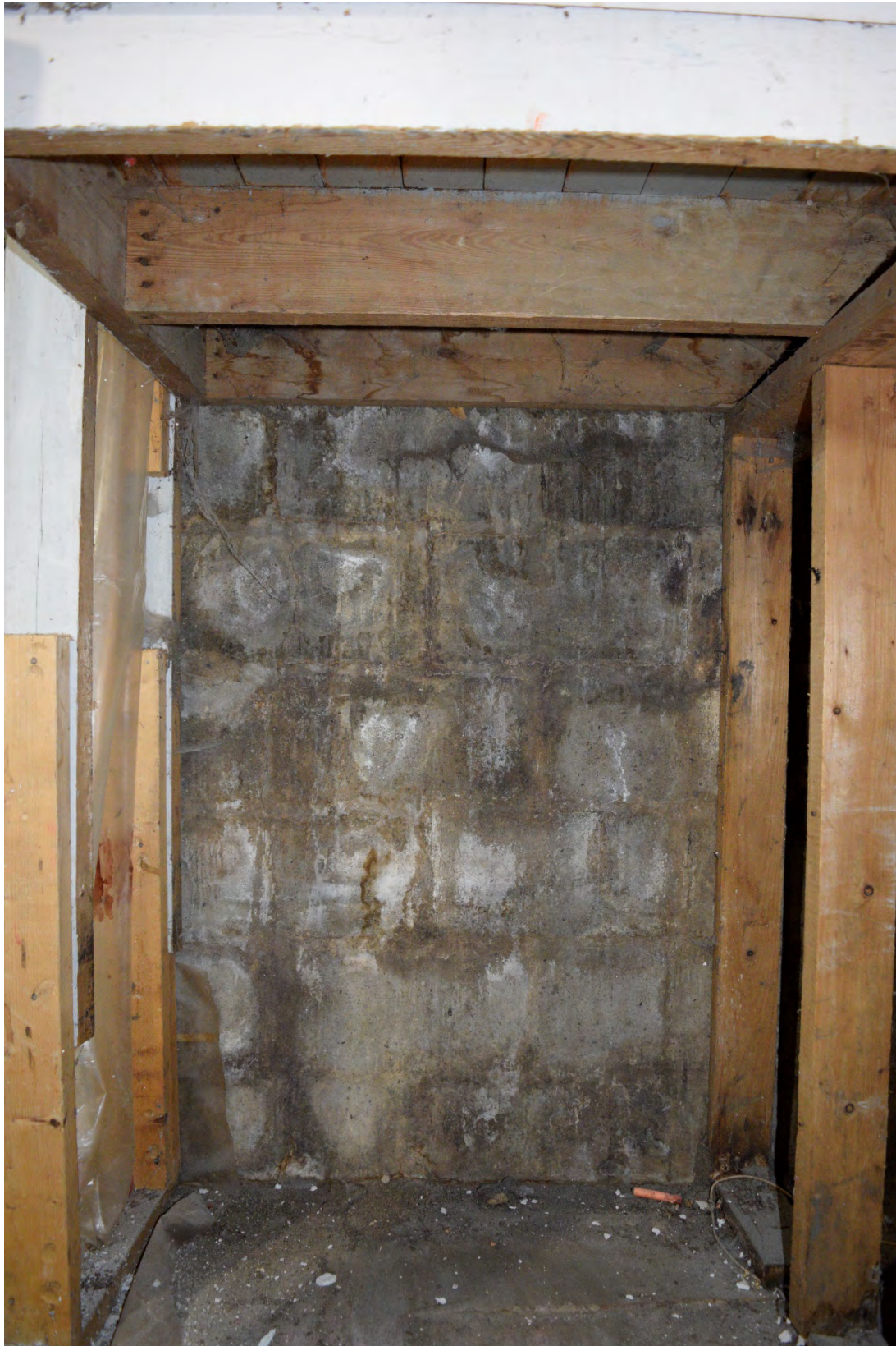
Image 26: Typical cement block foundation with poured concrete floor, facing east
