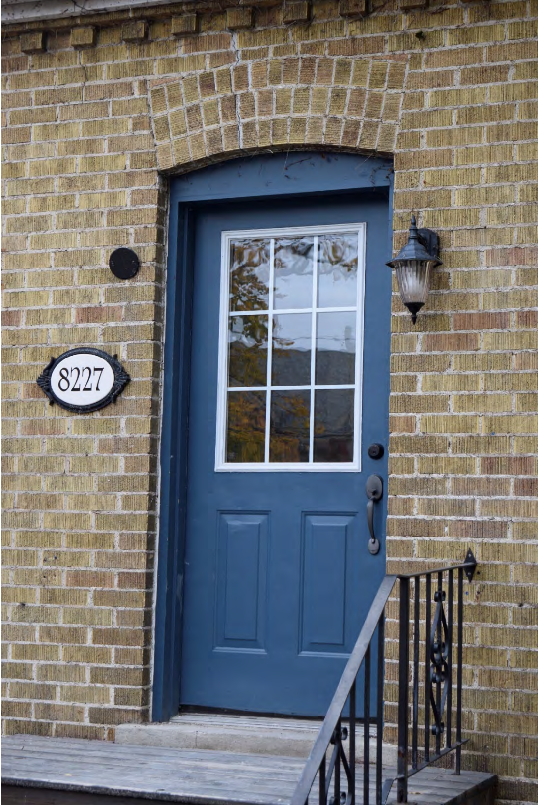
Image 10: Modern aluminum storm door at main entrance, note embellishment of segmental arch
