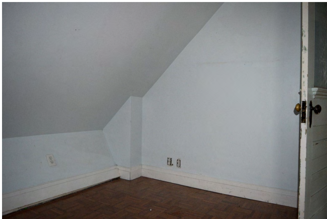
Image 22: West bedroom, note use of non original salvaged door and hardware, facing northeast
