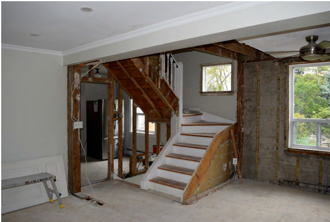
Image 13: Interior of residence showing original staircase, facing northeast
