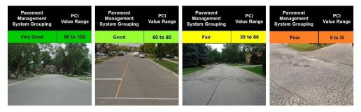
Figure 6-8: Images of Pavement Inspections Compared to Asset Management Condition Rating
