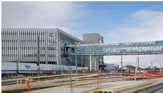
Construction Progress on Rutherford GO parking garage and pedestrian bridge
