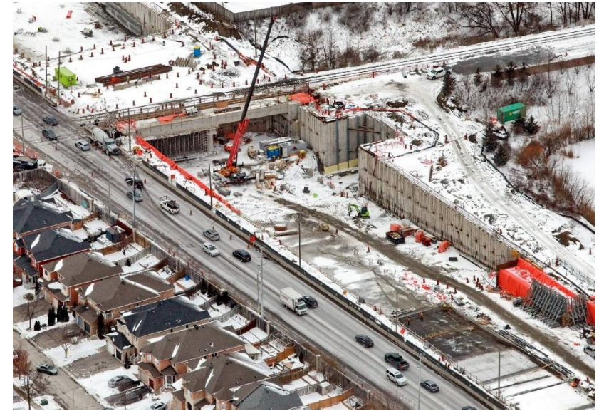
Ongoing Construction on Rutherford Road Grade Separation
