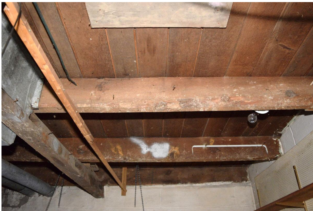
Figure 34: Planed wood joists and floorboards as seen from the Main Block basement.
