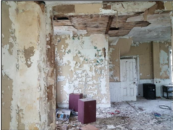
Figure 58: Looking west within the first floor of the existing building
