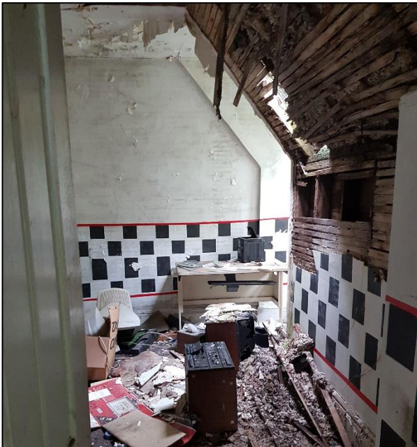
Figure 64: Looking north into the northeast bedroom at the second floor
