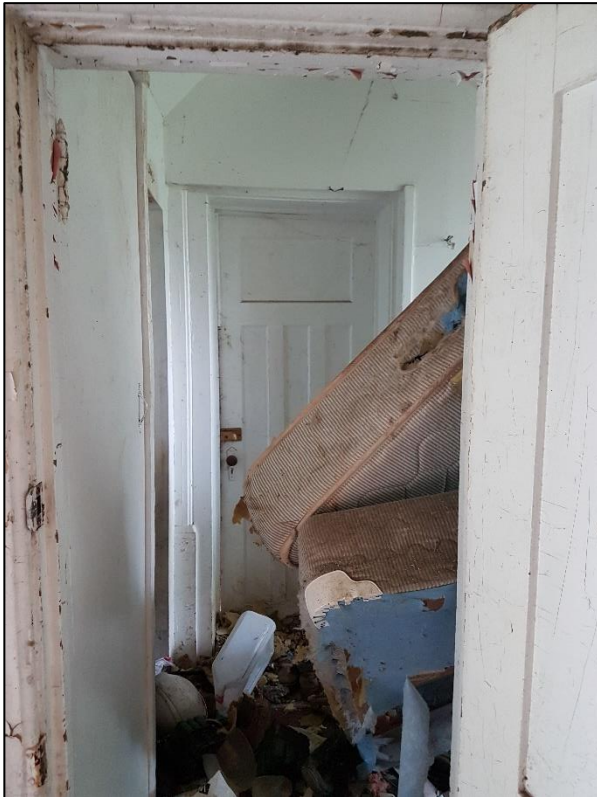
Figure 54: Looking west beyond the existing kitchen at the west end of the existing building (ASI 2019)
