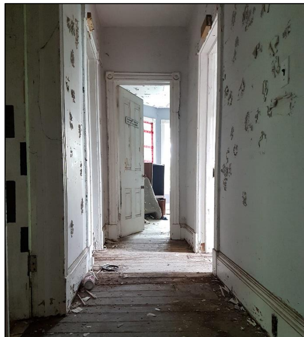
Figure 69: Looking east into the second-floor hallway
