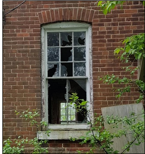
Figure 43: North elevation detail, showing the first-storey window opening
