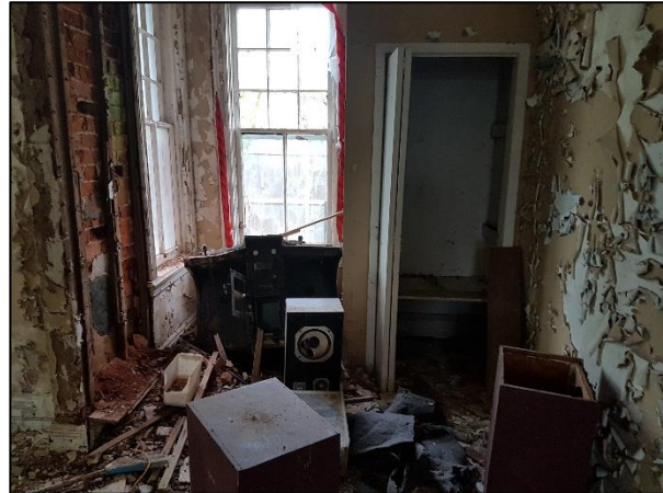
Figure 59: Looking south within the first floor of the existing building towards the south elevation
