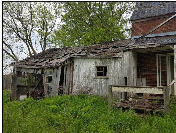
Figure 50: South elevation of the rear addition (ASI 2019)
