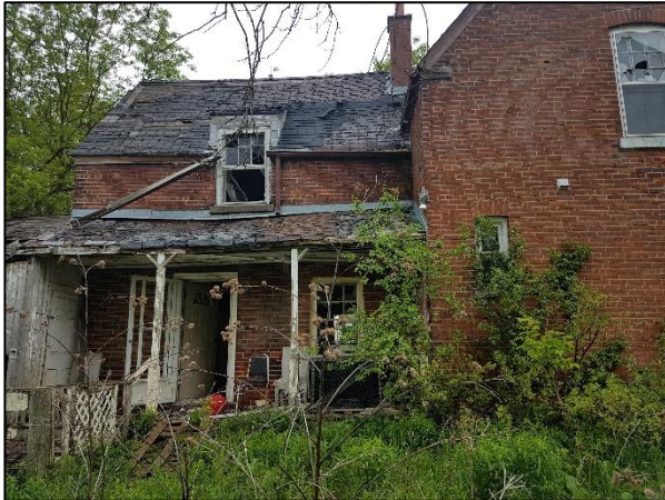
Figure 51: South elevation of the west wing (ASI 2019)
