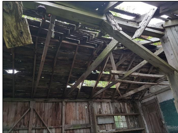
Figure 71: Existing roof of the rear wooden addition (ASI 2019)
