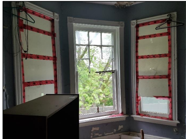
Figure 67: Bay windows within the east bedroom on the second floor
