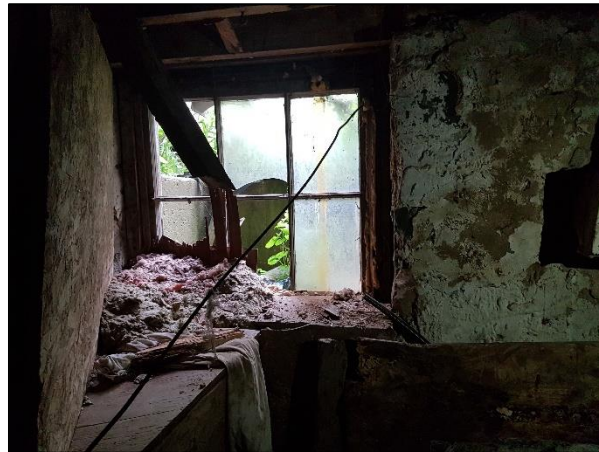
Figure 53: South elevation wall within the existing basement
