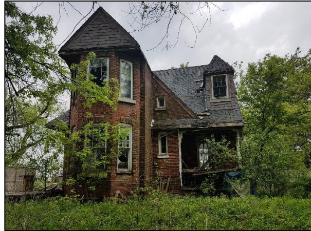
Figure 4: Existing residential building at 11110 Jane Street (ASI 2019)
