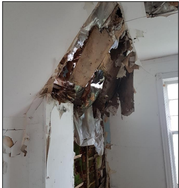
Figure 65: Sloped ceiling within the south bedroom at the second floor
