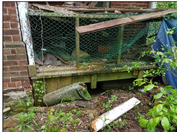
Figure 39: East elevation detail showing the enclosed space within the first-storey porch (ASI 2019)
