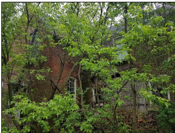
Figure 44: Partial north elevation of the existing building (ASI 2019)
