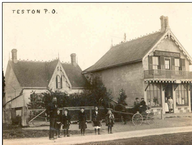
Figure 5: Post Office in Teston, Ontario, c. 1900 (City of Vaughan Archives 1900)
