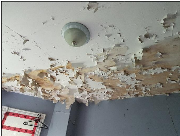
Figure 66: Ceiling within the east bedroom on the second floor
