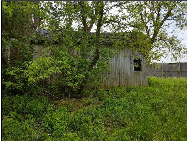
Figure 48: North elevation of the rear addition (ASI 2019)
