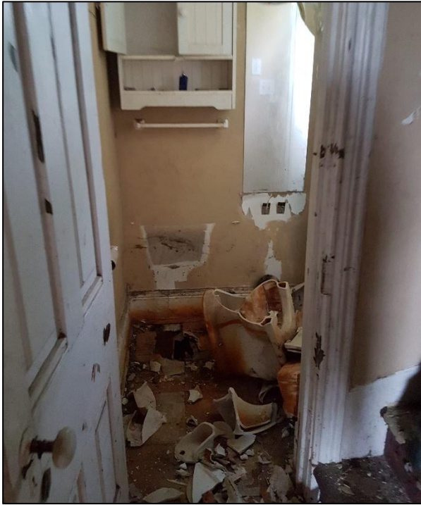
Figure 62: Looking east into the bathroom along the east elevation
