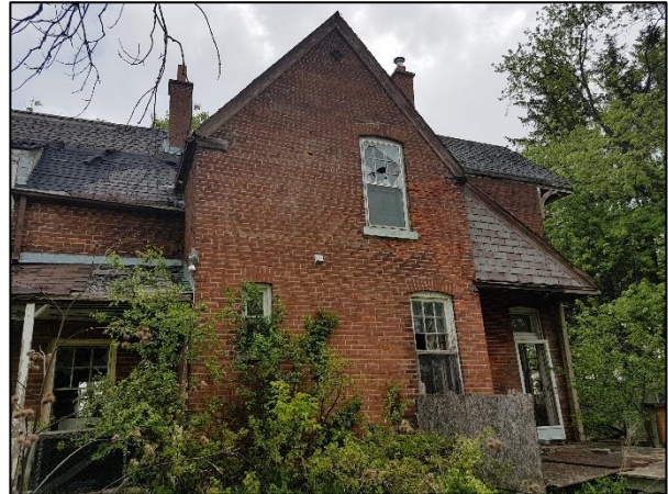
Figure 52: East portion of the south elevation (ASI 2019)
