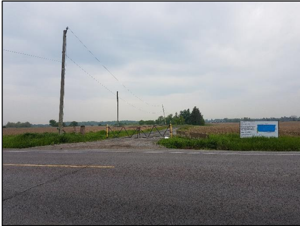
Figure 3: Subject property at 11110 Jane Street, looking west into the property from Jane Street (ASI 2019)
