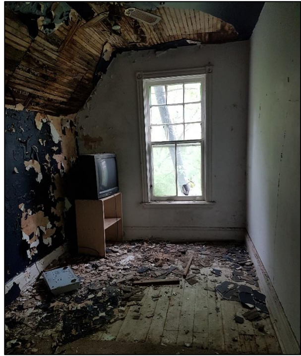
Figure 63: Looking north into the northwest bedroom on the second floor
