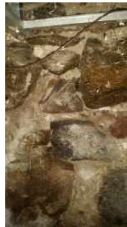
Interior view of stone / rubble foundation
