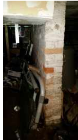
Brick load bearing wall
