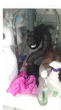
S-Trap drain configuration under main floor bathroom sink
