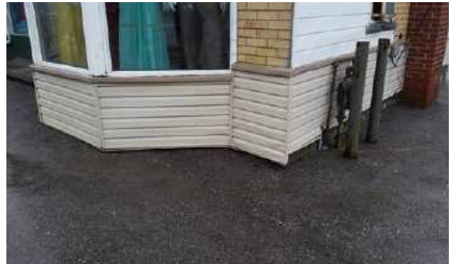
Siding extends to grade at front of dwelling
