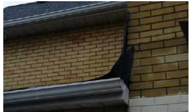
Improper wall flashing
