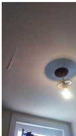
Light fixture with missing cover
