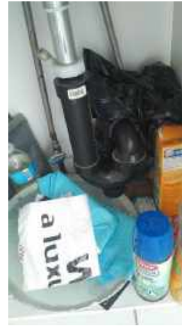
S-Trap drain configuration under second floor bathroom sink
