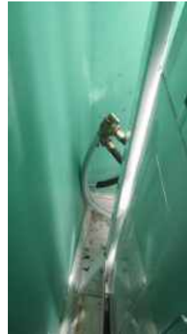
PEX lines for washing machine
