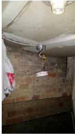
Smoke detector in basement hanging from junction box
