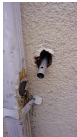
Damaged / perforated downspout
