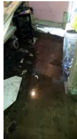
Standing water at rear portion of basement
