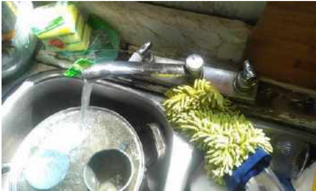
Sink Faucet mounted on section of wood over counter
