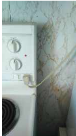
Stove outlet also used for small appliance
