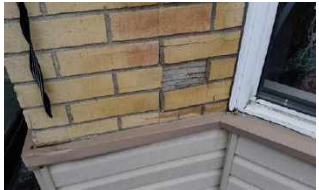
Close-up view of failing brick tile. Cracked and spalling of surface / cement substrate.
