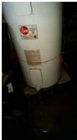
Electric HWT on concrete blocks in basement
