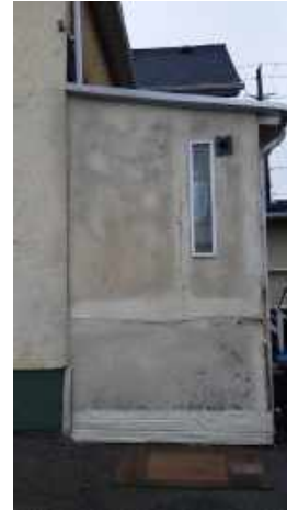
Rear wall of porch enclosure. Dark areas indicate water penetration into substrate material.
