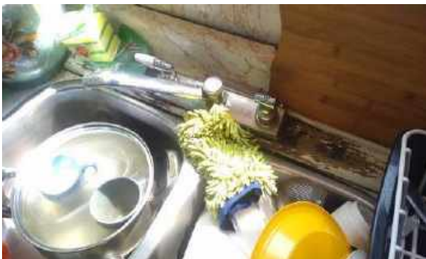
Counter deteriorated around sink area
