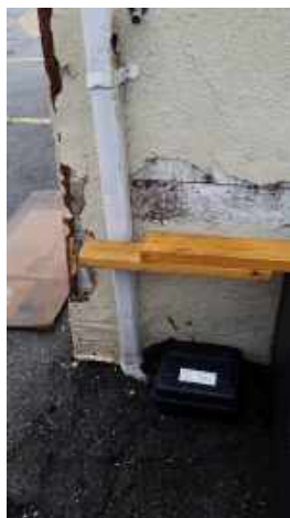
Downspout noted as extending into below grade drain pipe
