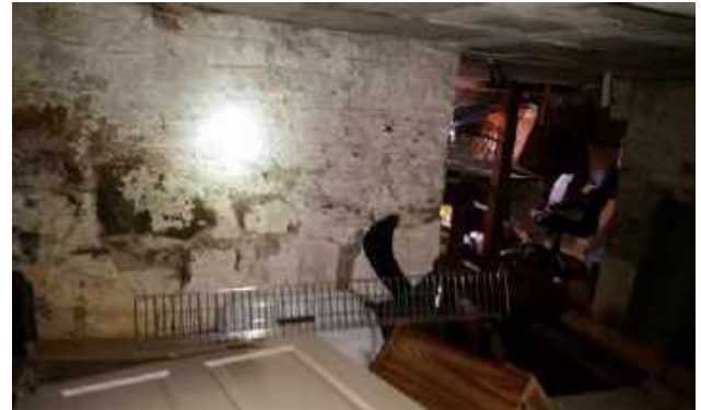
Water stained / damaged foundation wall
