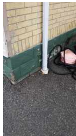
Downspout below grade discharge
