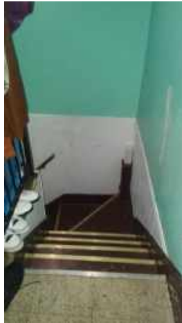
Section of stairs with missing handrail
