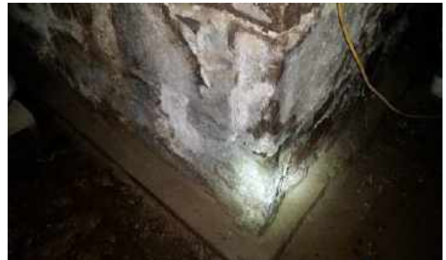
Significant amount of efflorescence on inside of foundation wall caused by moisture migration through the wall
