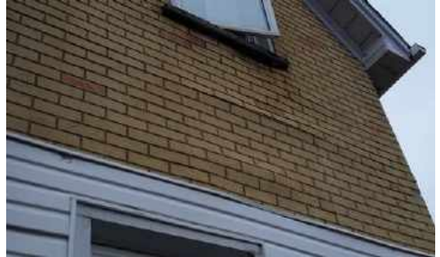
Wall area below window sill failing. Brick tile finish is buckling.
