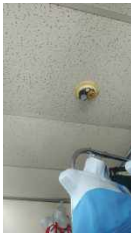
Main floor inoperative smoke detector
