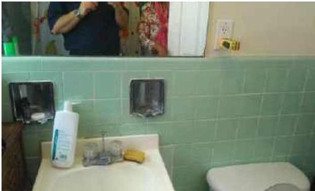
Non GFCI outlet (also open ground condition noted)
