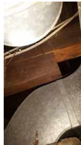
Cracked / compromised floor joist
