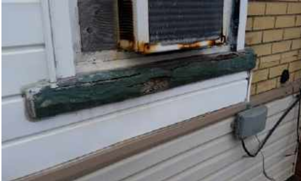
Deteriorated cement window sill has no capacity to keep water out of wall
