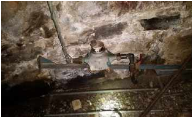
Main water shut-off valve and meter
