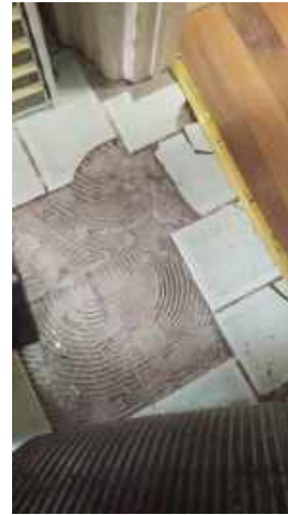
Cracked / broken floor tile
