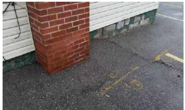
Brick chimney extends below grade
