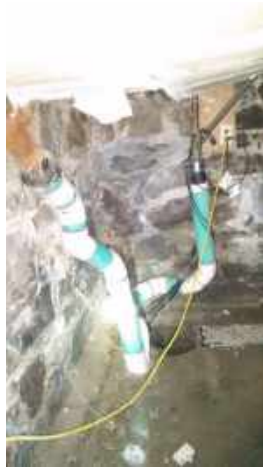
Cast iron and brass connection to newer PVC type drain pipe in basement
