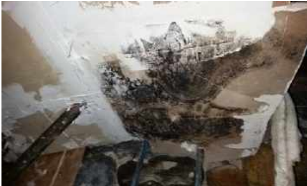
Mould growth noted on underside of ceiling drywall
