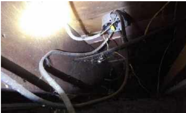
Old wires spliced with new in open junction box
