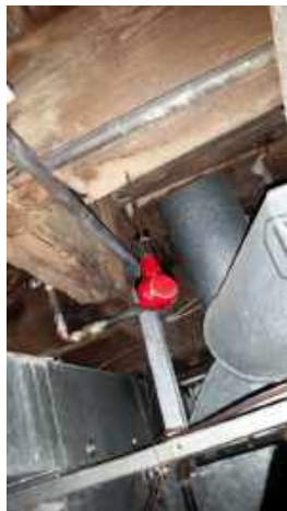
Visible wood joists not structurally compromised
