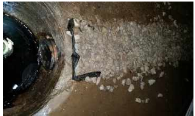
Trench / drain pipe leading into sump pit
