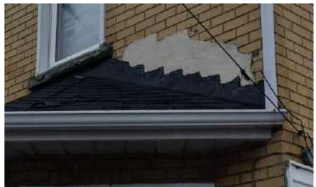
Parged wall above flashing
