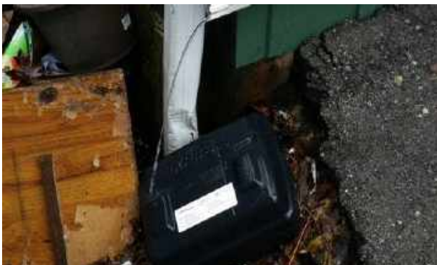
Downspout at front of building discharging at grade
