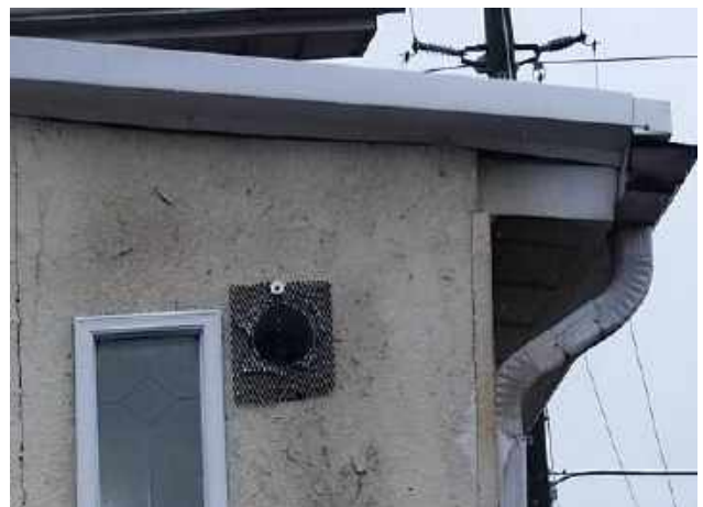
Exterior unprotected dryer vent
