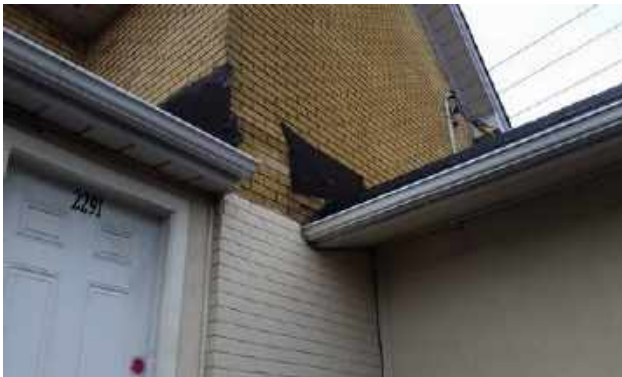
Improper wall flashing at lower roof plane
