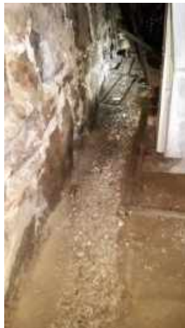
Perimeter trenching along inside of foundation wall
