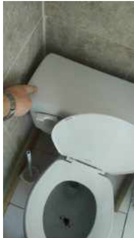
Loose toilet in second floor bathroom
