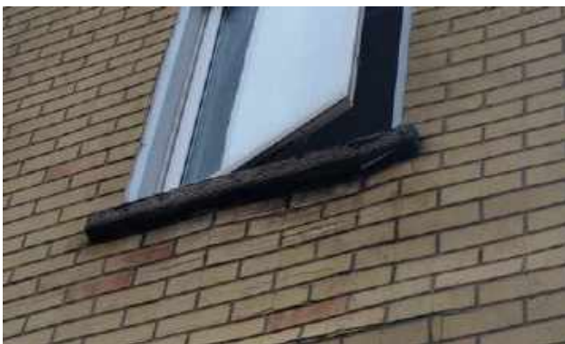
Badly deteriorated window sill on second floor level
