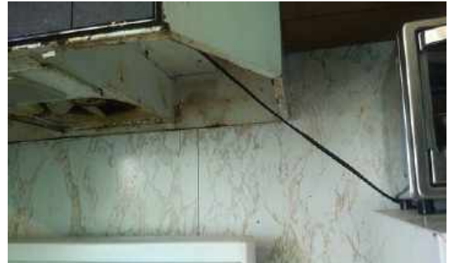
Kitchen fan connection to outlet
