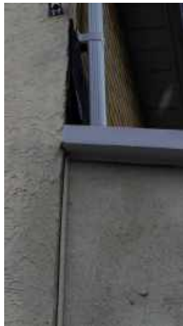
Gap in flashing at wall noted above roof
