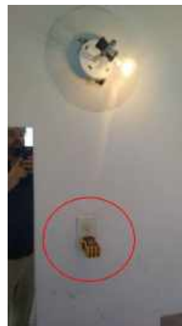
Inoperative outlet (also exposed bulb above)
