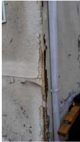
Damaged stucco corner of wall
