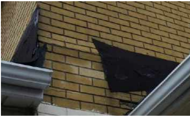
Brick tile finish noted as buckling at corner of building.
