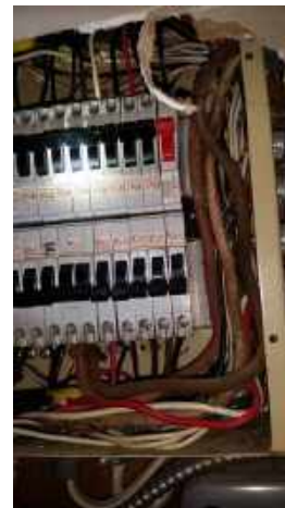
Old cloth sheathed wiring noted in panel servicing the stove still in place
