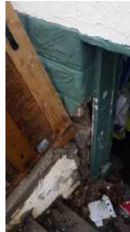
Cracked / broken foundation wall at basement walk-out
