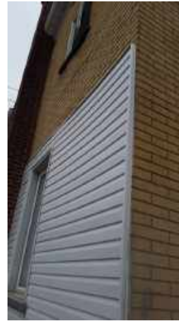
Indiscriminate wall area with siding applied over brick tile.
