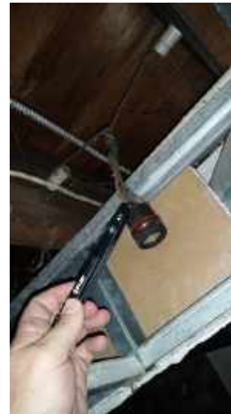
Old active knob and tube wiring
