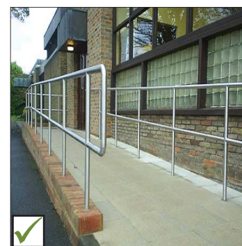
Figure 7c: Handrail Returns to Floor
