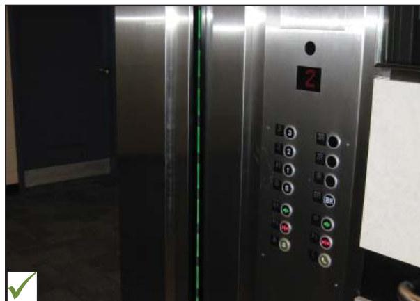
Elevator sensor door and floor registration buttons.
