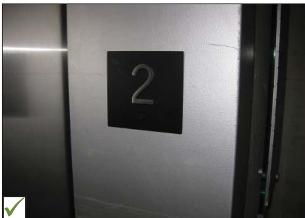
Tactile elevator car identification sign.
