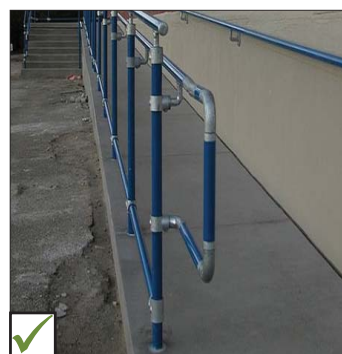
Figure 7b: Handrail Returns to Wall
