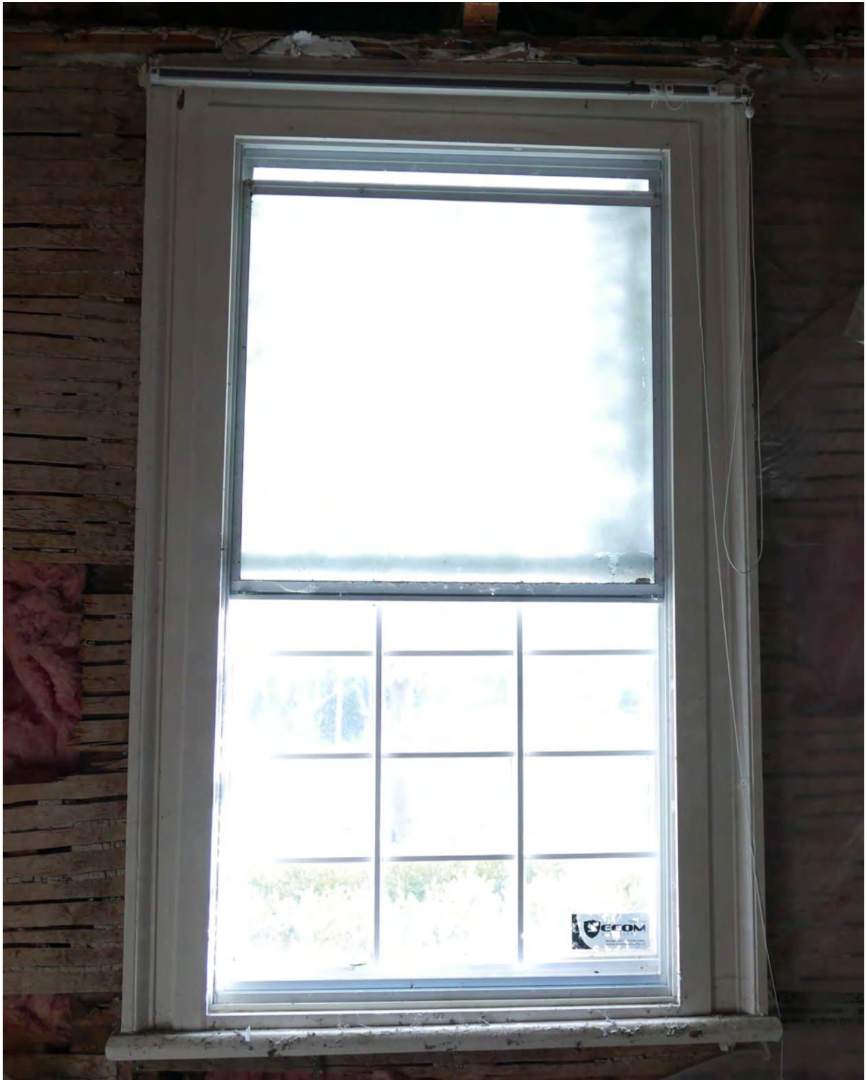
Figure 26: Historic casings remain at the Main House's interior windows, despite being obscured by storm widnows. Profiles differ slightly on the ground floor windows (CBCollective, 2020).
