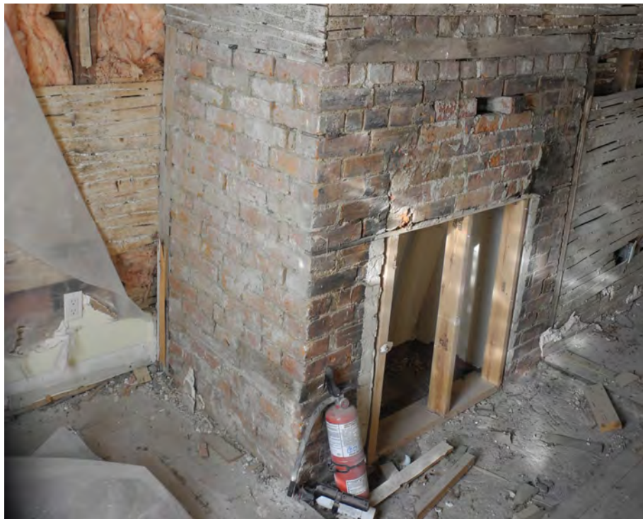
Figure 19: Masonry chimney structure, built entirely within the timber structure of the Main House ( CBCollective, 2020 ).
