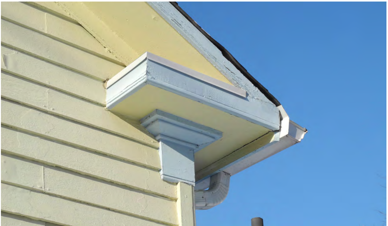
Figure 17: Detail of fascia and soffit at north-east gable return. The historic fascia board is deteriorated, and that of the return is poorly detailed. Note the oversized fascia board on the north elevation ( CBCollective, 2020 ).
