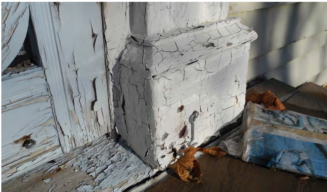
Figure 24: Door surrounds are in good shape overall, with paint failure most pronounced at the pilaster bases (CBCollective, 2020).
