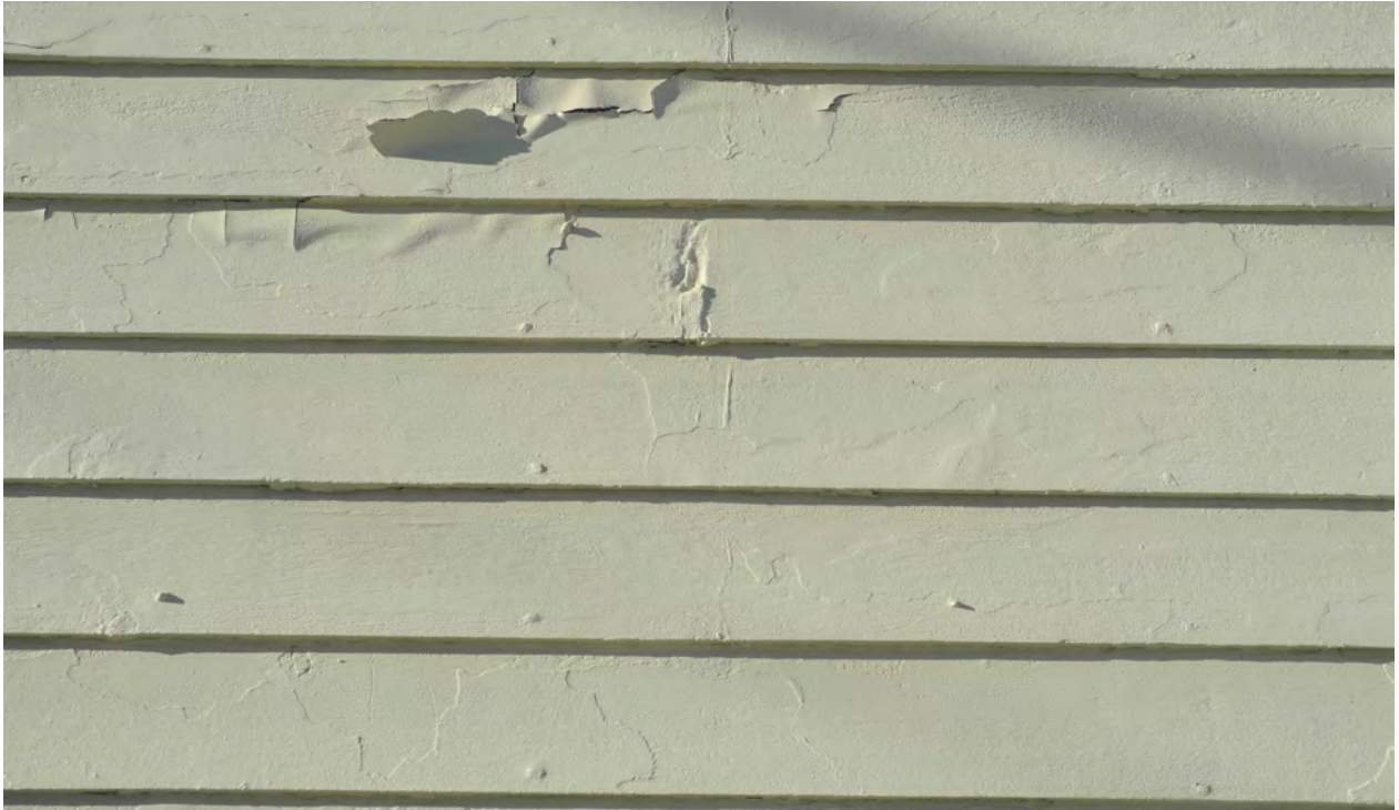
Figure 7: Detail of typical cladding, with nails, paint failure, and previous paint visible (CBCollective, 2020).
