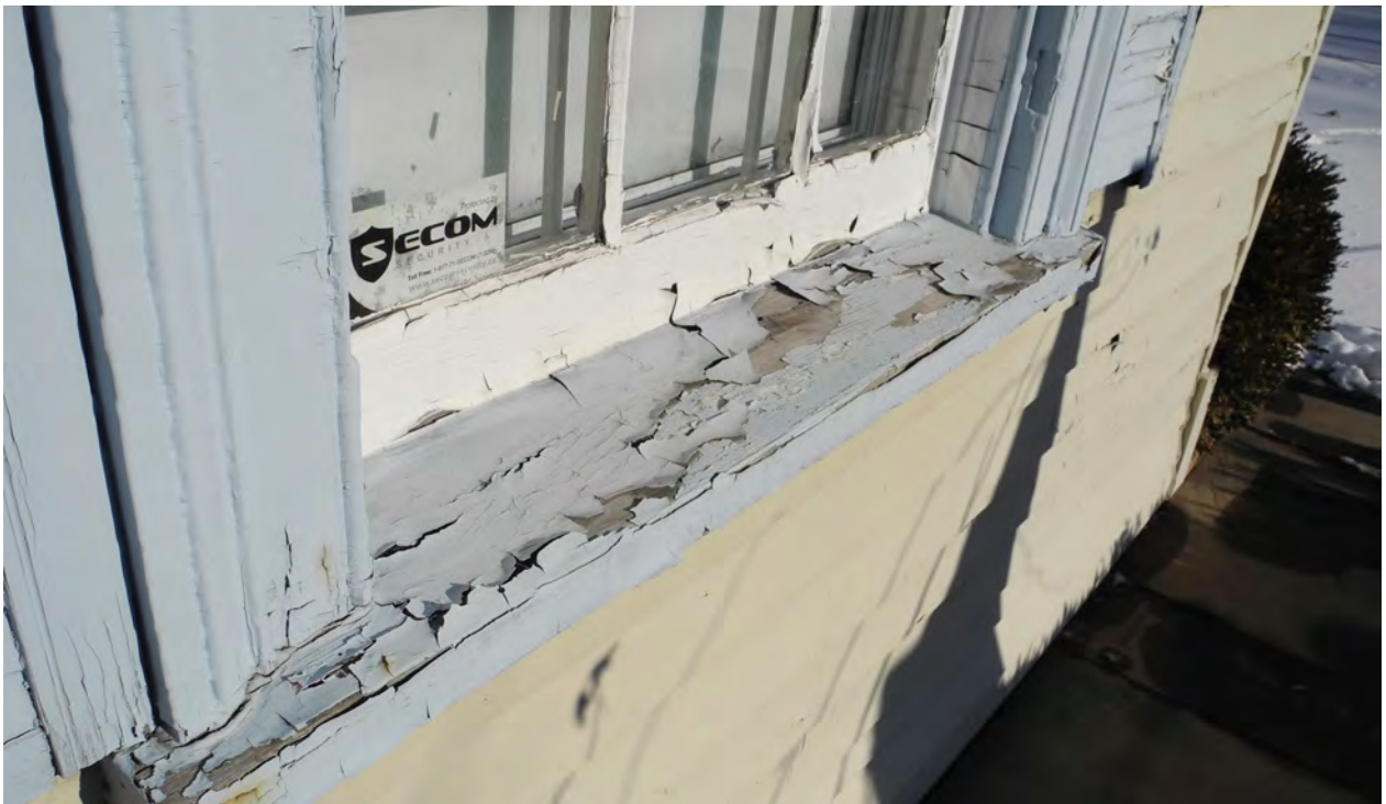
Figure 23: Detail of severe paint failure on sills, and at the bottom of the casings. Note mortises for earlier functional shutters on the far casing ( CBCollective, 2020 ).
