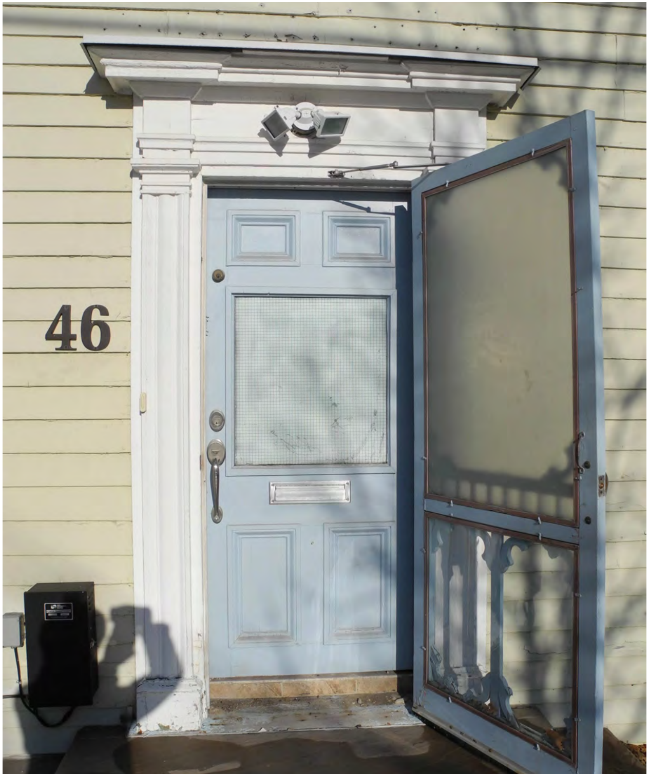
Figure 9: Main House front door showing modified panel door and screen door set within classical surround ( Michael Scott Architect, 2020 ).
