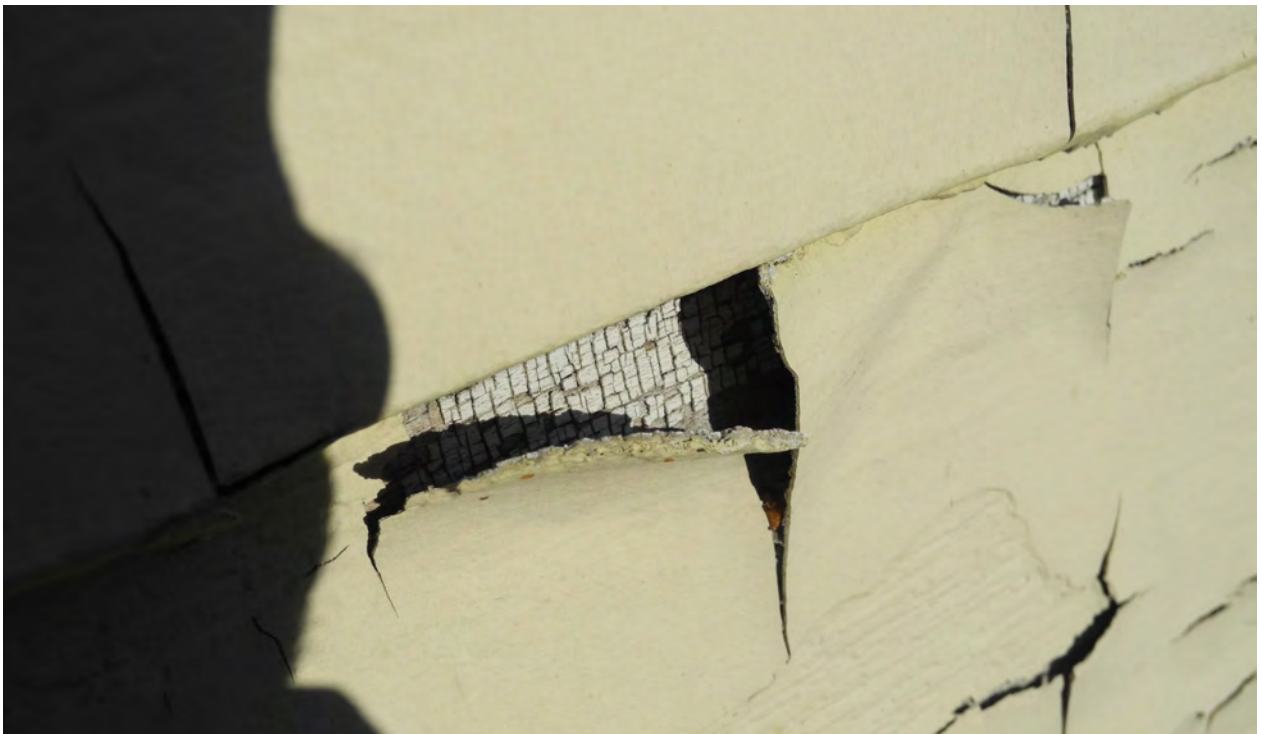
Figure 13: Detail of cladding, showing advanced paint failure revealing revealing earlier finishes beneath ( CBCollective, 2020 ).
