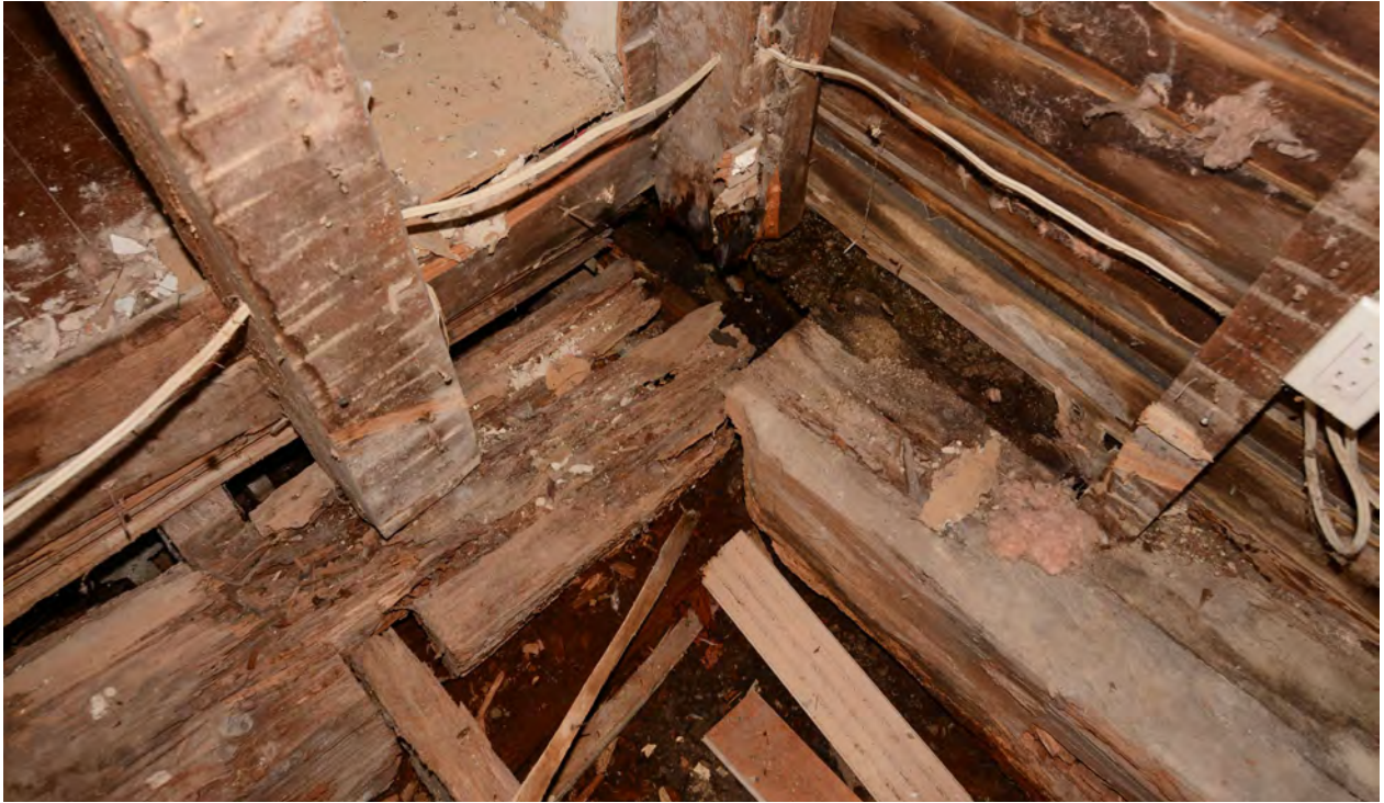
Figure 10: Detail of heavily decayed sill plate at north-east corner of Main House. Deterioration has caused sill plates to separate from each other as well as vertical posts, and drop several inches ( Michael Scott Architect, 2020 ).
