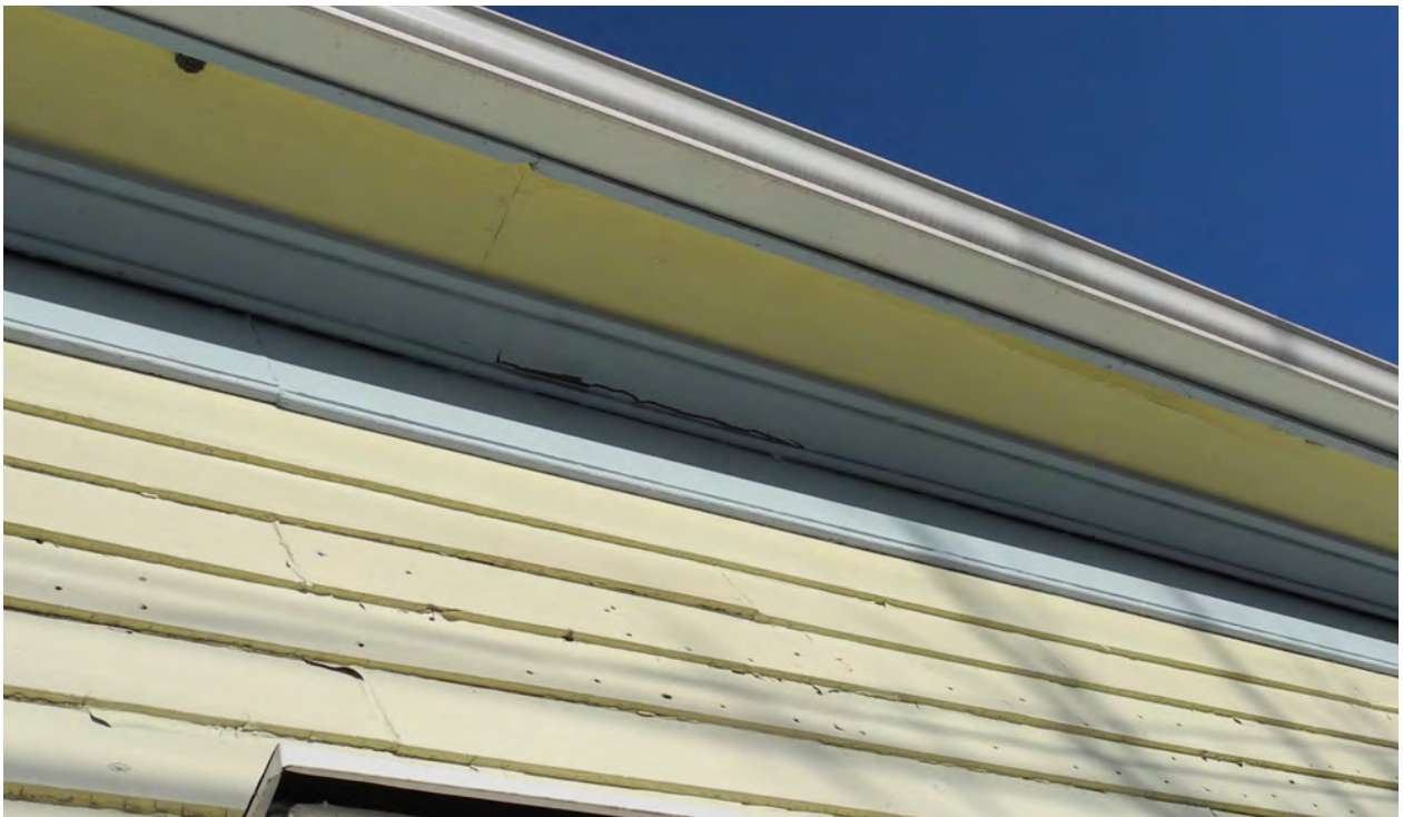
Figure 15: Detail of frieze board and mouldings above front door, showing good overall condition with paint failure (CBCollective, 2020).
