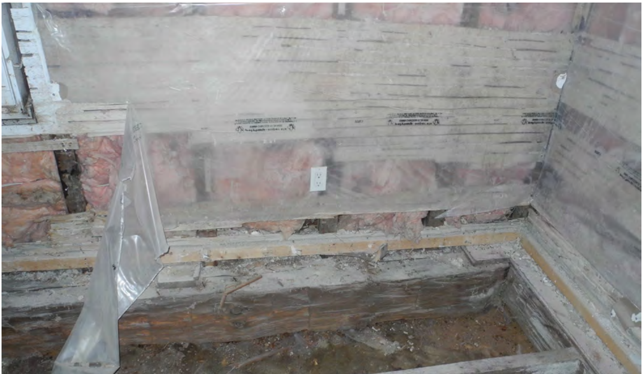
Figure 6: South end of the Main House's east wall, showing sill plates set directly on the soil (CBCollective, 2020).
