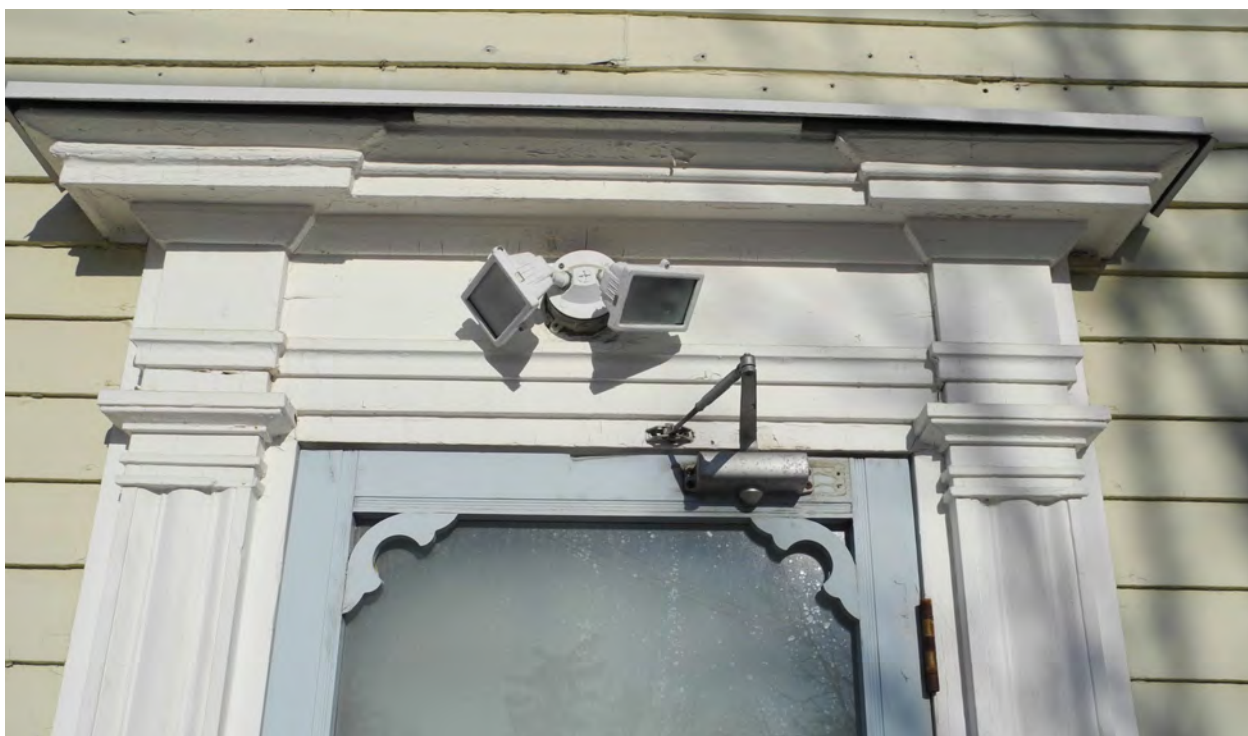
Figure 25: Flashing over the door surround is in fair condition, but it obscures the plan of the surround, effectively diminishing the detail's legibility (CBCollective, 2020).
