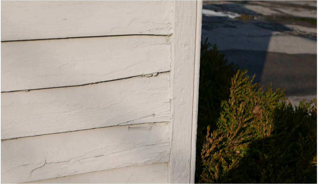
Figure 14: Detail of Main House's south-east corner, showing cracked cladding related to nail locations (CBCollective, 2020).
