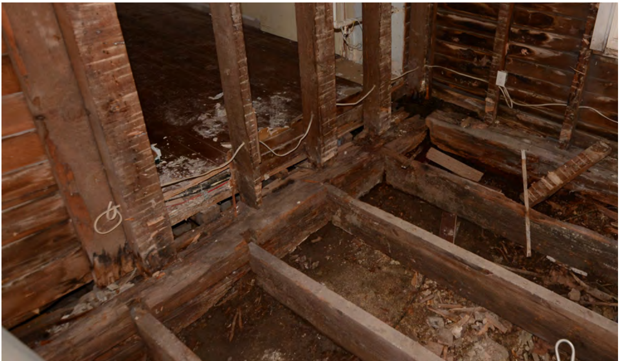
Figure 11: Detail of Main House's north wall, showing floor joists and posts mortised directly into the sill plates ( Michael Scott Architect, 2020 ).
