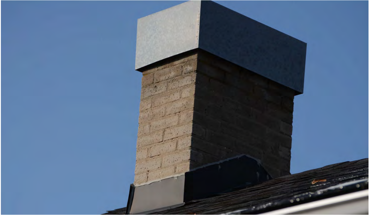
Figure 20: Detail of exterior chimney showing masonry, galvanized cap, and flashings all in good condition ( Michael Scott Architect, 2020 ).
