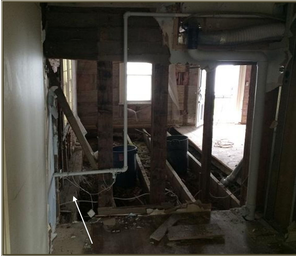
5.4.13 Southward view toward (and through) front wall of house showing joists in soil and heavy timber sill indicated by white arrow, 15 November 2017.
