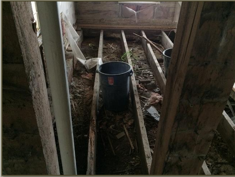
5.4.7 View of ground floor joists, probable original mass, in relation to soil, 15 November 2017.
