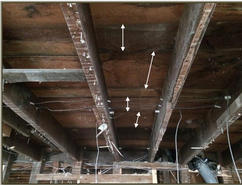
5.4.6 Second floor ceiling joists showing lath marks. Note width of sub-floor boards indicated by white arrows, 15 November 2017. Wider boards were used more frequently as the supply of lumber wasn't considered scarce or threatened.
