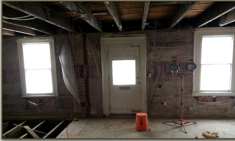
5.4.3 View of interior of front (south-facing) wall of probable original mass, 15 November 2017. Note compressed space between top of windows & door and upper floor joists.
