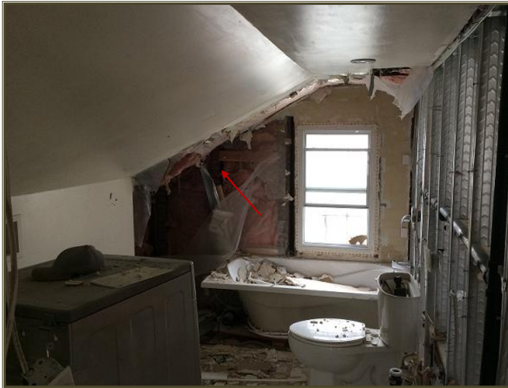
5.4.20 Northern-most window in east wall of upper half-storey, probable original mass,, 15 November 2017. Red arrow indicating 2" x 4" stud with lath marks.
