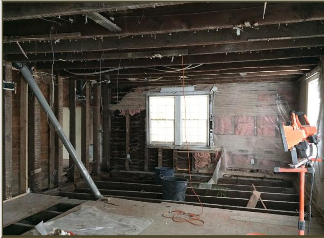
5.4.5 Eastward view across ground floor space, southern-most (original) mass showing 6" x 6" and 2" x 4" framing, heavy timbers sill with floor joists in contact with soil, 15 November 2017.
