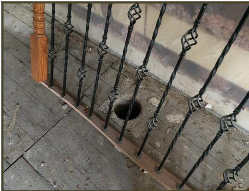
5.4.12 Detail of disused floor chase as indicated by white arrow, Figure 5.4.11, above, 15 November 2017.
