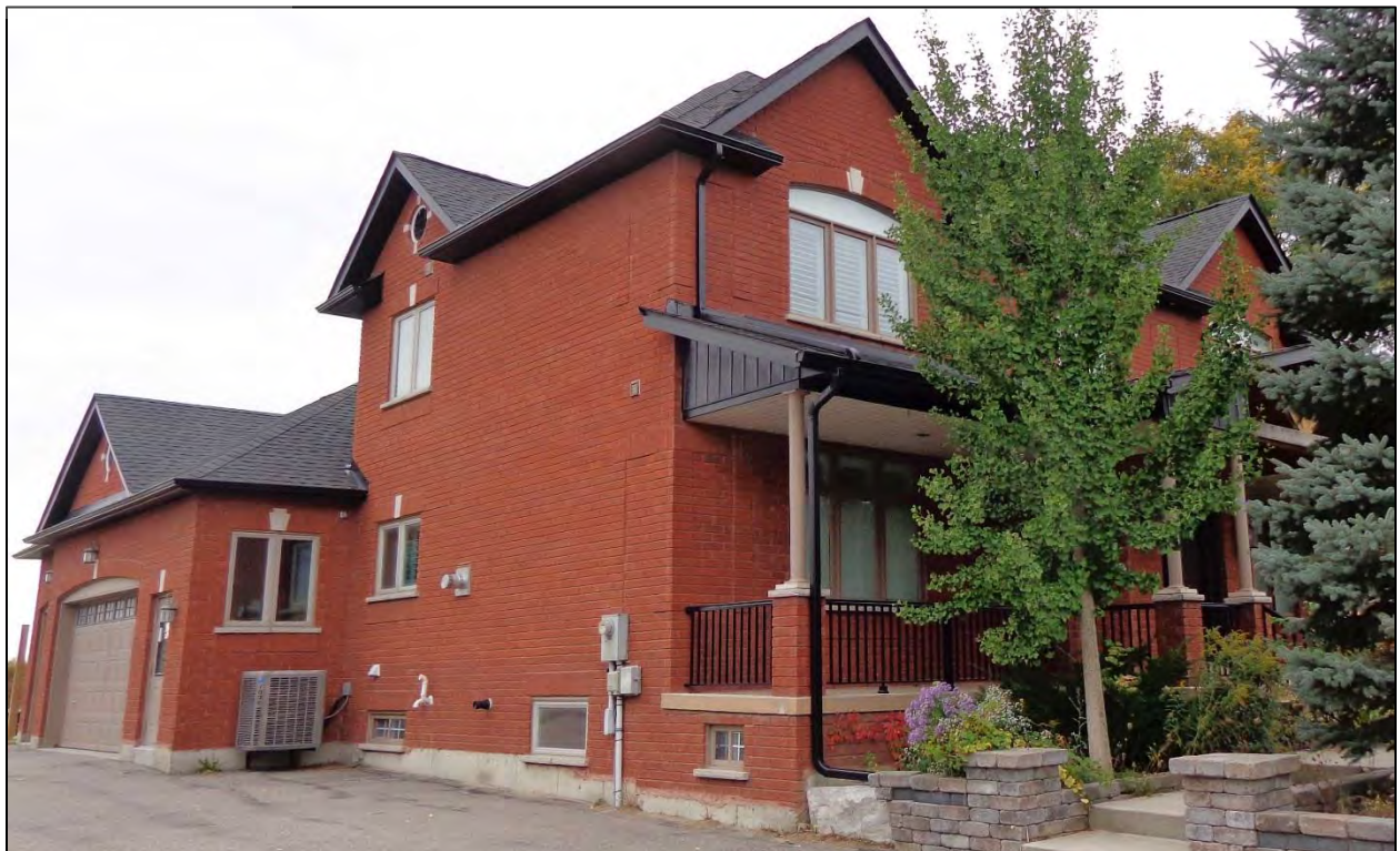
South and East Elevations
