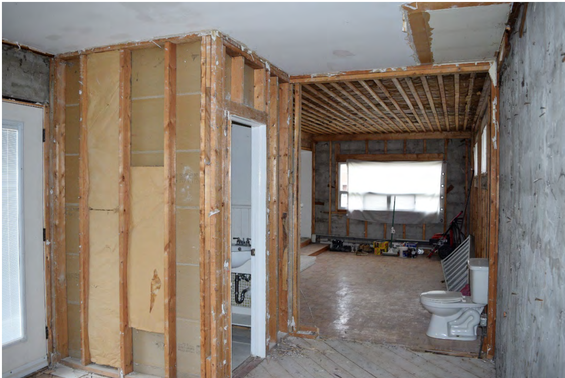
Image 17: Interior of north addition, facing west
