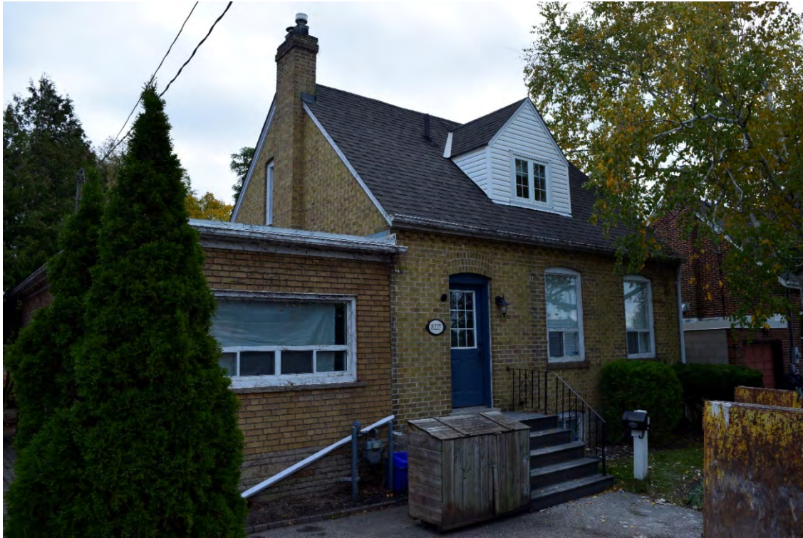
Image 3: Front façade of 8227 Kipling Avenue, facing east-southeast
