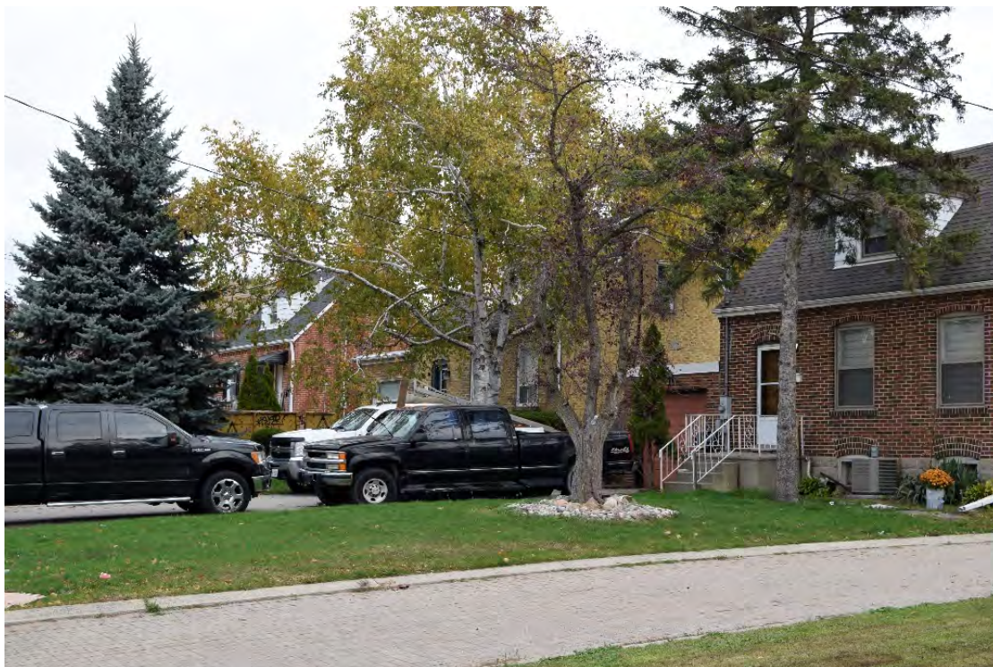
Image 2: Garage addition on 8221 Kipling Avenue, Subject Property is visible to the left.
