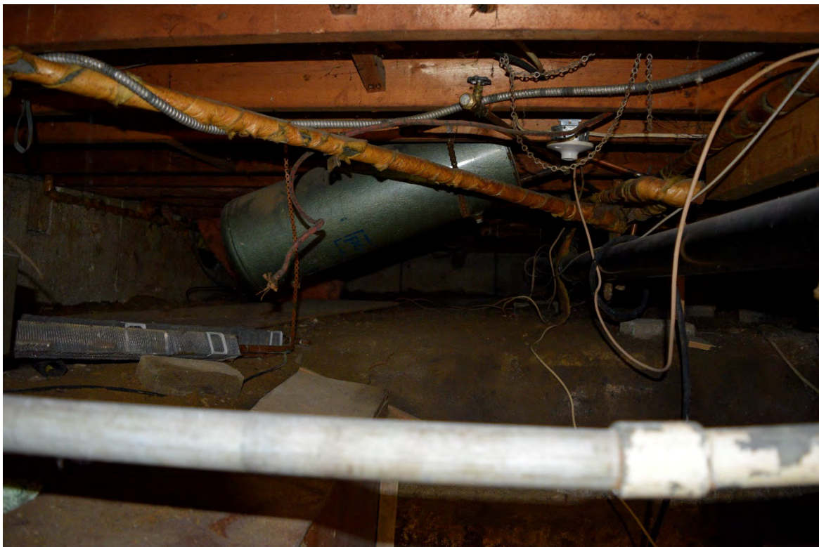
Image 25: Crawl space under north addition, facing west
