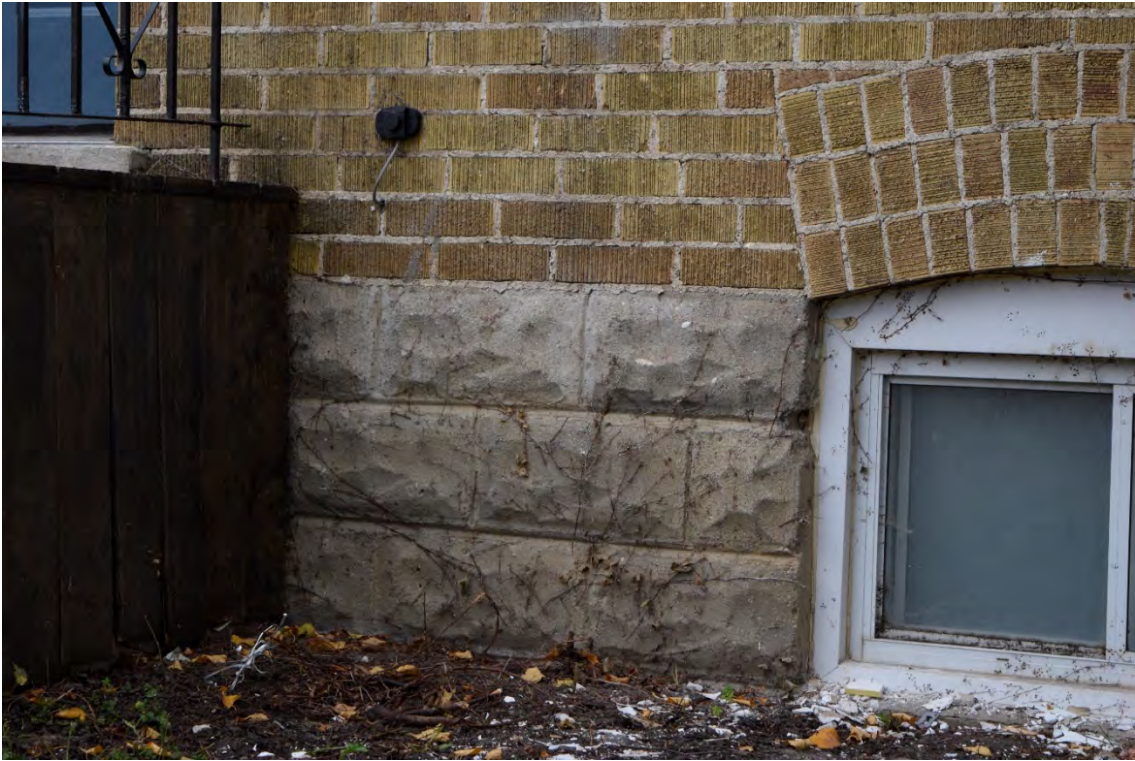
Image 8: Rusticated cement block used for foundation of original structure
