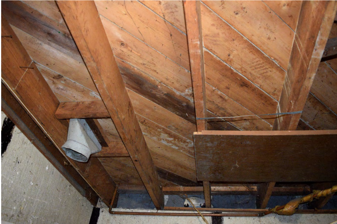
Image 24: Typical floor joists and subfloor construction, joists are 2" x 6" set 16" on center
