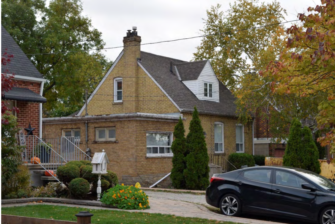
Image 5: North face of Subject Property, note difference in brick finish of northern addition, facing south-southeast
