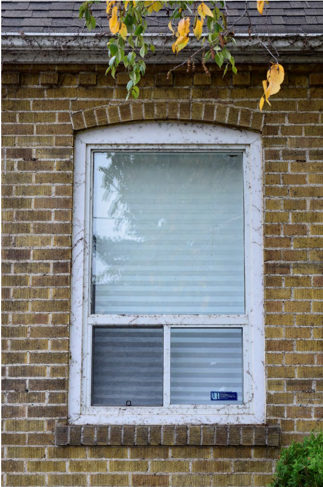
Image 9: Example of typical vinyl window, note segmental arch at head of window and brick lug sill.
