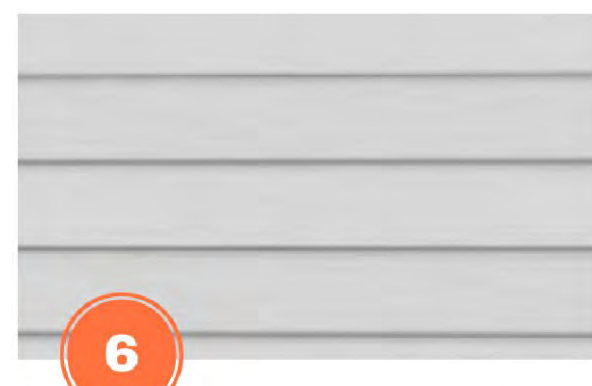
6 Existing Siding Colour: White
