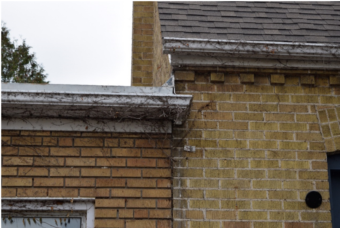
Image 7: Close up of seam occurring between north addition and original structure, note brick dentate at eve.
