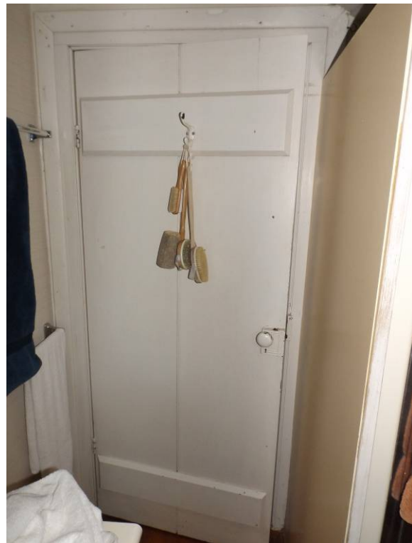
Figure 28. Second floor, very wide plank door. The bathroom and the tiny bedroom are the only two rooms that retain these doors.
