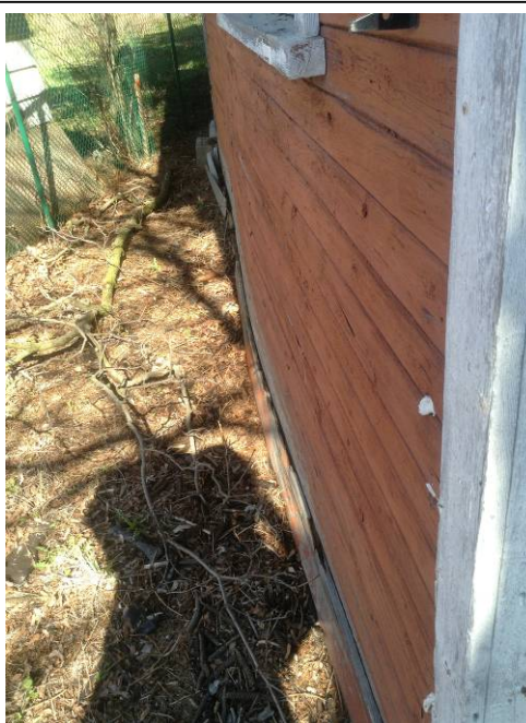
Figure 13. There is a significant bow at the base of the west wall near the south corner.
