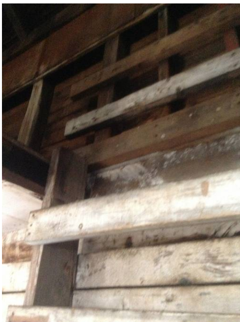
Figure 12. Top of the ladder shows large header on top of lower plank on plank wall, supporting frame of loft level. It's possible that the loft was added later.
