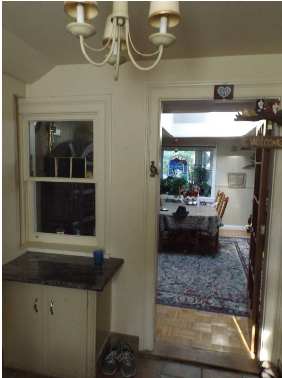
Figure 20. Looking from the entry door into the central 1-storey dining room. We believe this window and door openings were once in the exterior wall of the tail of the house.
