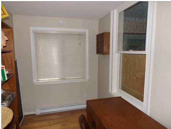
Figure 21. Ground floor, verandah, looking south. The window on the right looks into the front room. We believe it is in an original exterior opening, left from the previous version of the house. Being interior, it didn't require a thermal upgrade when the last alterations occurred. This window and the matching one behind us are the only surviving exterior elements of the mid-20 th century iteration of the building.
