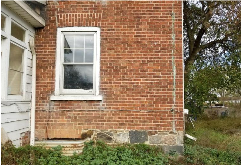
Figure 22: Detail of Flemish Bond and coursed rubble foundation on the west façade of the Main Block.
