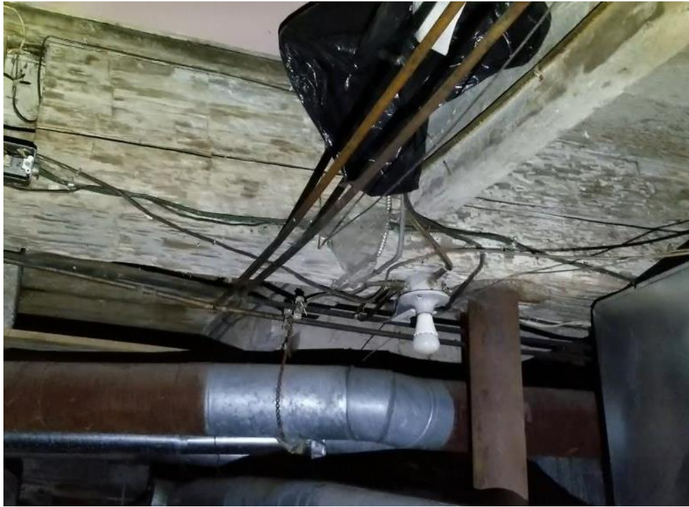
Figure 47: Close up of the summer beam running east-west across the basement ceiling.
