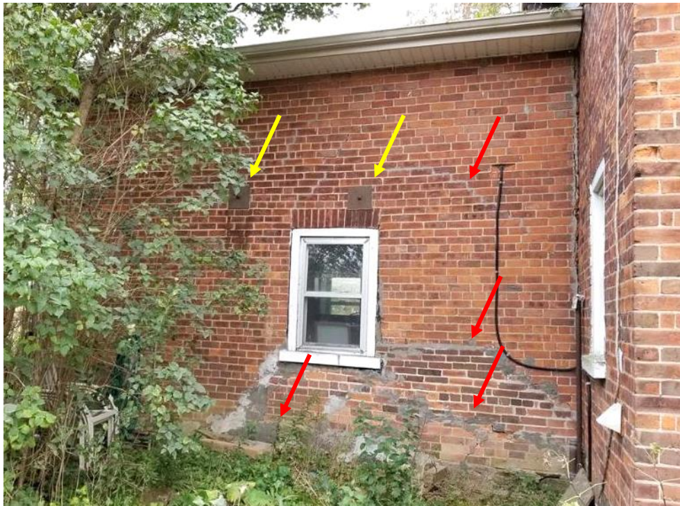
Figure 50: Extensive damage and repair to the north wall (red). Note the metal rods to secure the wall (yellow).
