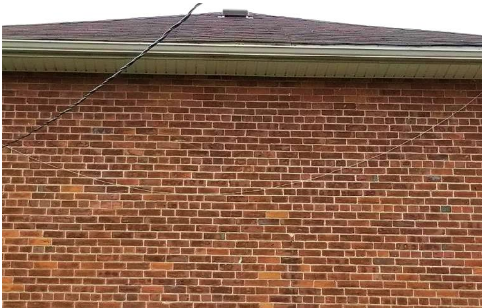
Figure 23: Detail of Common Bond on the north façade.
