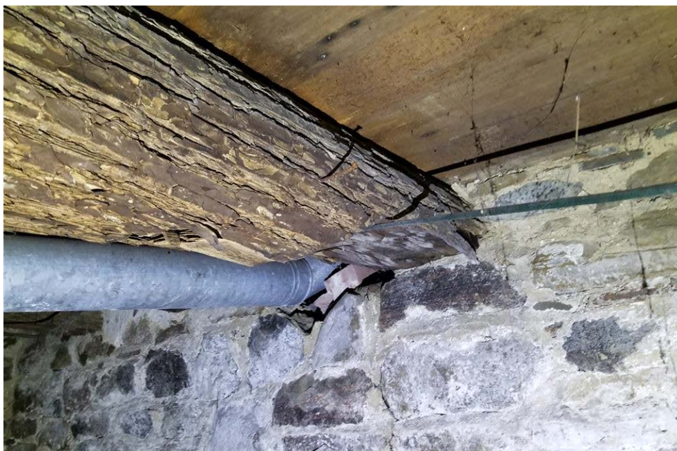
Figure 16: Example of overhead sleeper.
