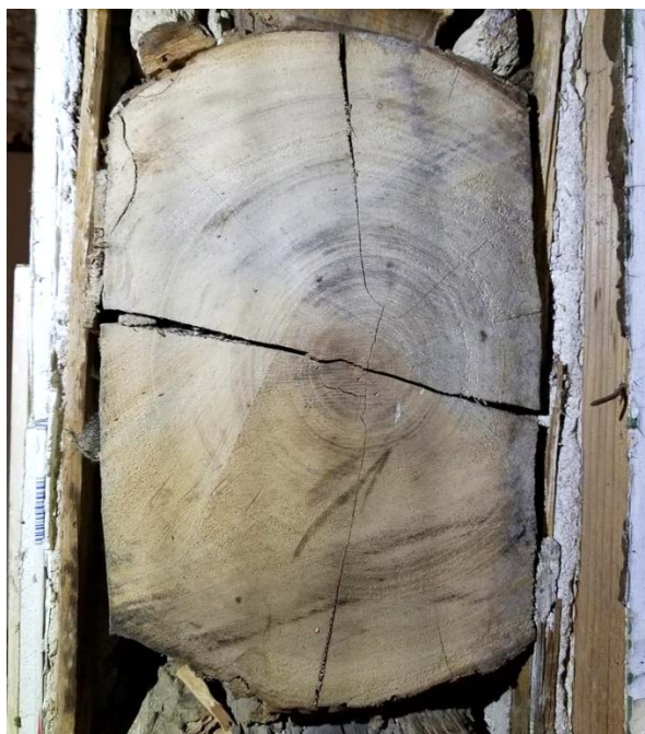
Figure 7: Cross-cut saw marks.
