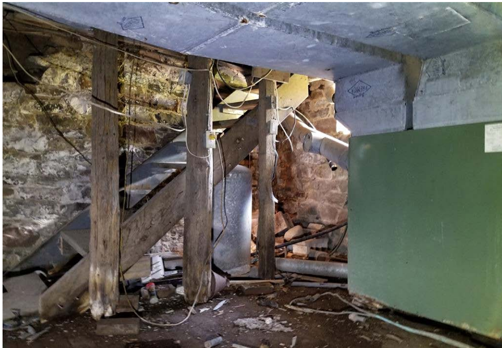
Figure 13: Stairs in the southeast corner of the basement, with three support posts.
