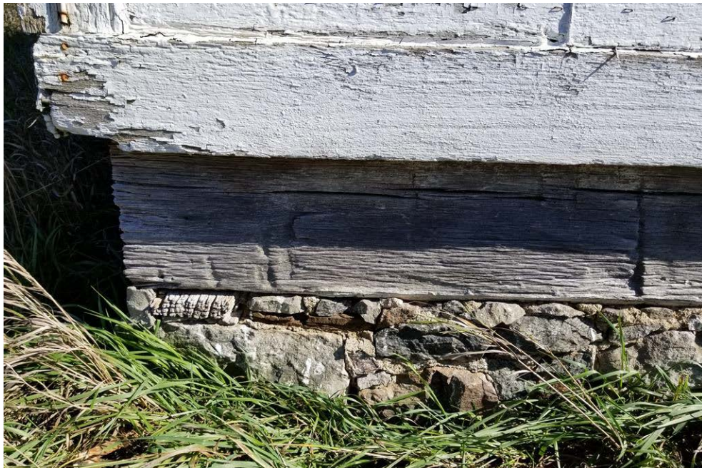
Figure 4: Coursed rubble foundation of the Main Block.
