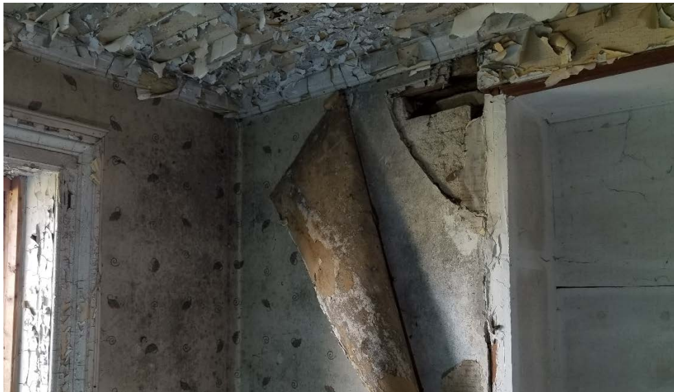
Figure 22: Bricks visible behind wallpaper and plaster, southeast corner of the ground floor room.
