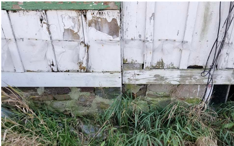
Figure 21: Joint visible in foundation in East Wing and Main Block.
