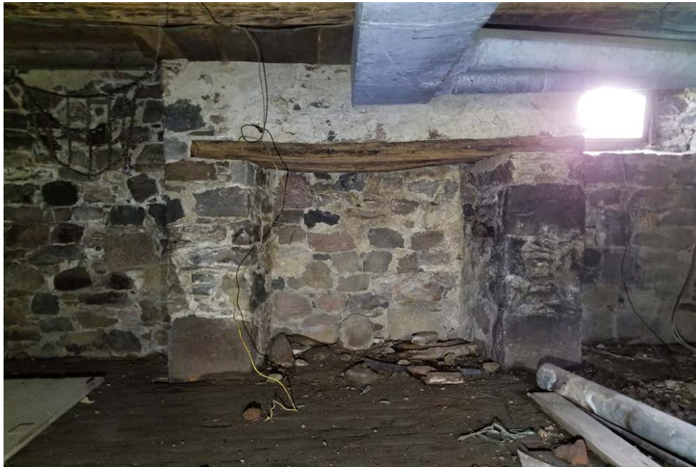
Figure 15: Fireplace at north end of basement, with wood lintel.
