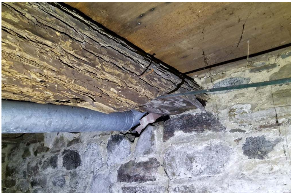
Figure 16: Example of overhead sleeper.
