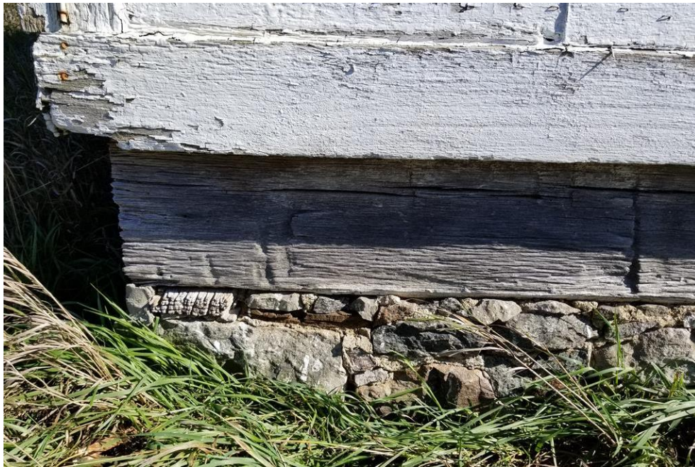
Figure 21: Coursed rubble foundation of the Main Block.
