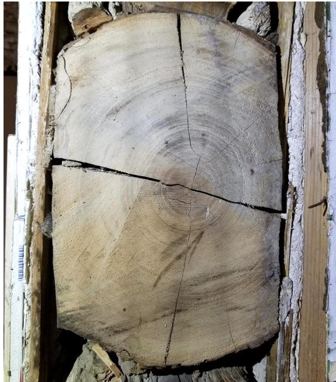
Figure 32: Cross-cut saw marks.
