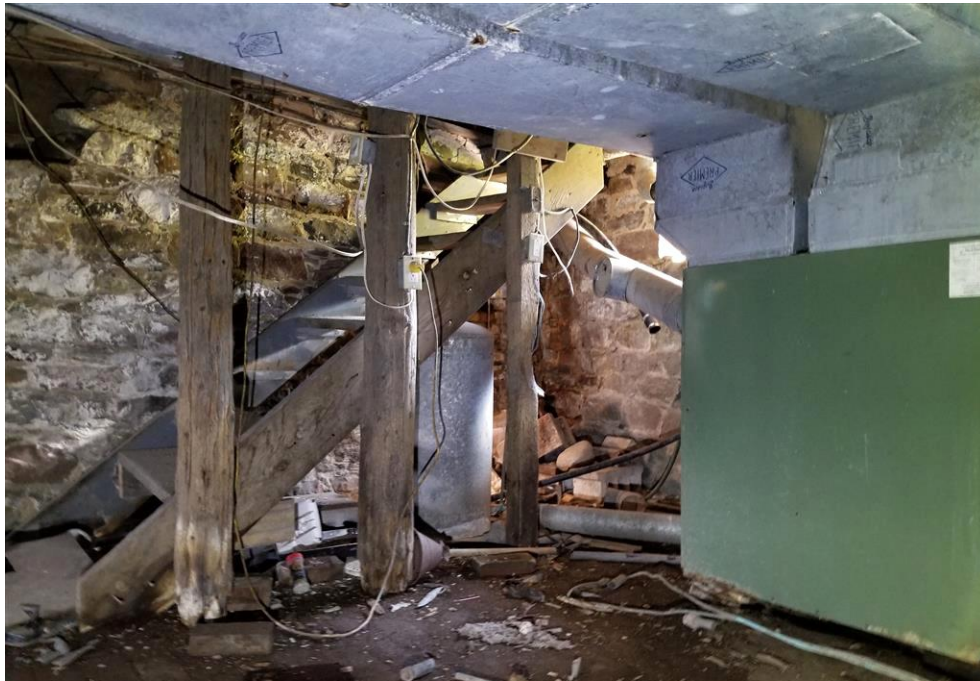
Figure 38: Stairs in the southeast corner of the basement, with three support posts.
