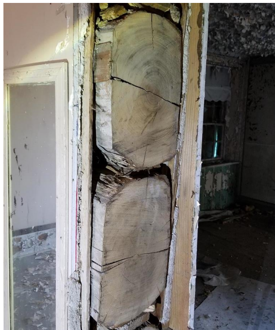
Figure 31: Interior east log wall on the Main Block.
