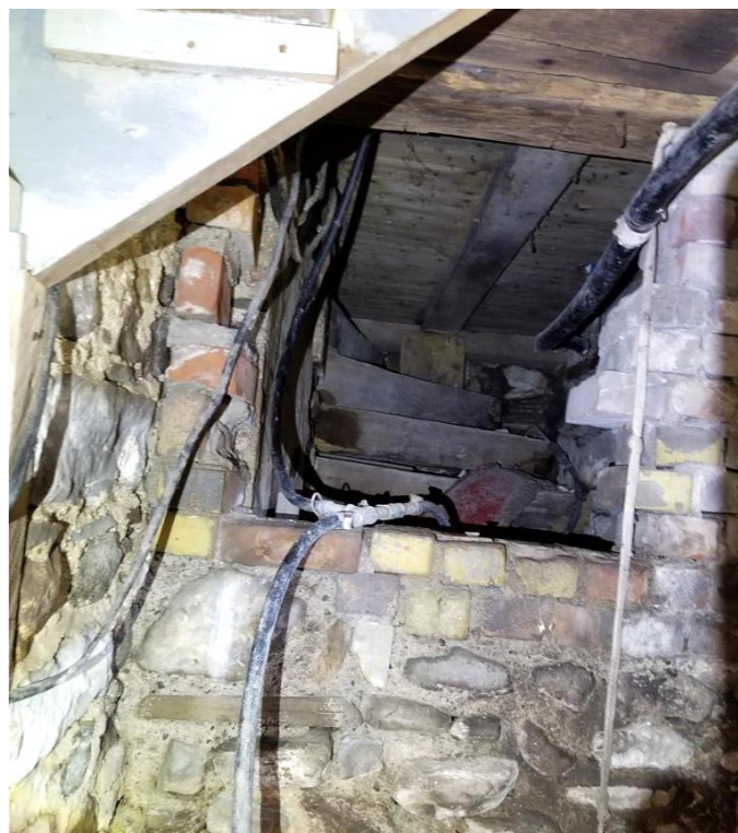
Figure 42: Crawlspace in east wall of basement. Crawlspace is below the East Wing.
