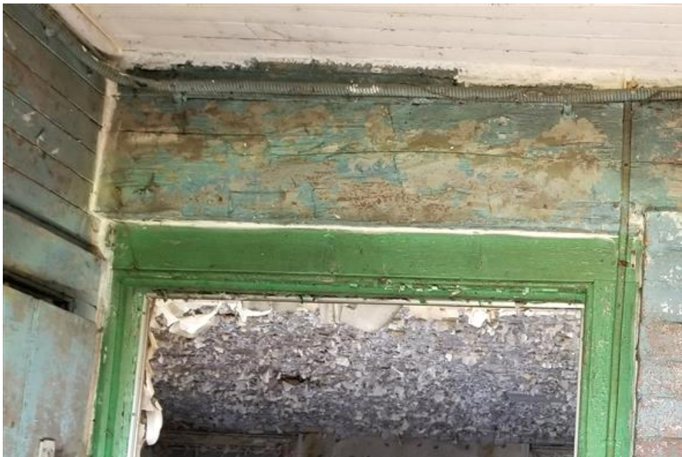
Figure 65: Adze marks on wood lintel above the door to the South Addition.
