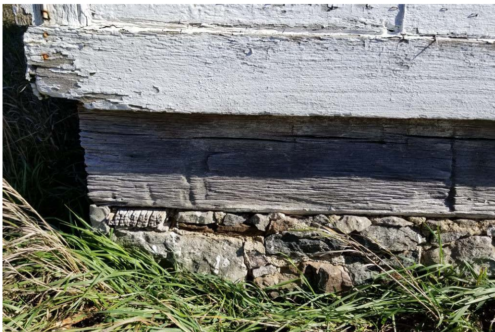
Figure 4: Coursed rubble foundation of the Main Block.
