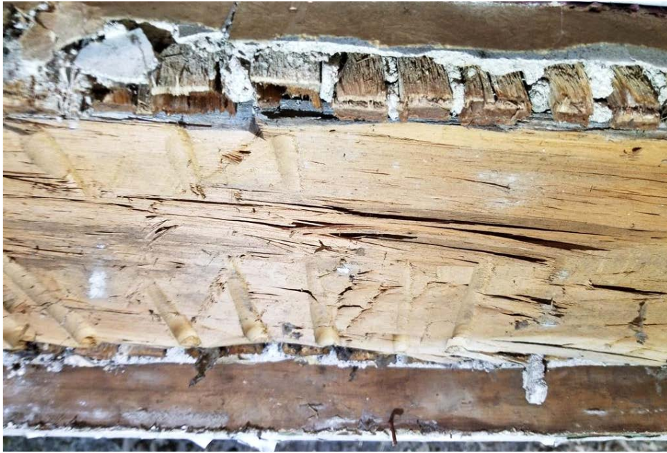
Figure 8: Detail of top of the doorway, showing split log and vertical lath and plaster.
