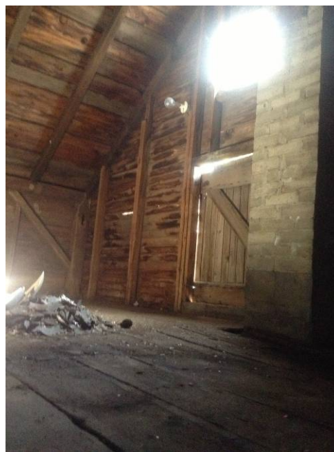
Figure 14. The upper level is barn framed with corner posts, braces, and infill studding. Brick chimney is visible on the right. It is at the centre of the south gable. Water damage to the sheathing boards is visible. Daylight is coming through one gap to the left. Note brick chimney to right of loading door.
