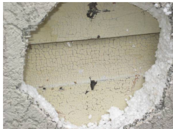
Figure 43. Cut out of recent EIFS stucco over Styrofoam, showing underlying wood drop channel shiplap siding. We believe the nail holes once secured the insulbrick siding.
