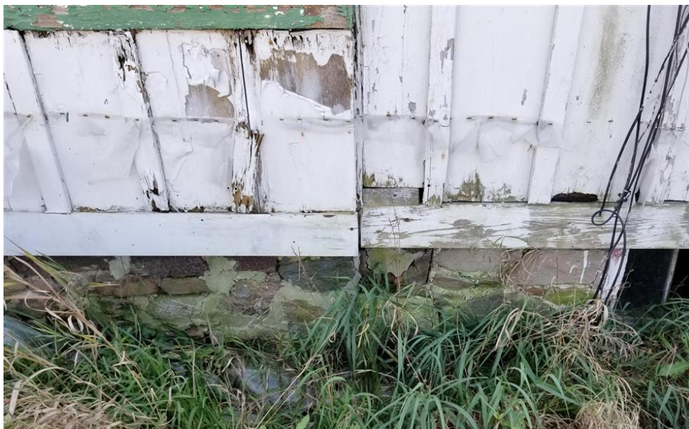
Figure 49: Join visible in foundation in East Wing and Main Block.
