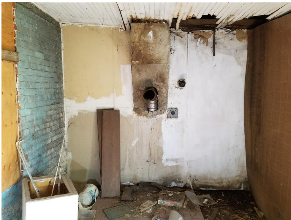
Figure 63: East wall of the South Addition, with stove flashing and wood panelled ceiling.
