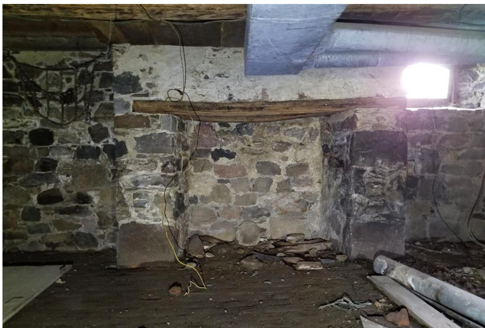
Figure 40: Fireplace at north end of basement, with wood lintel.
