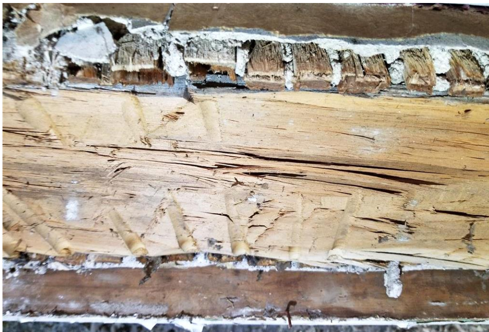
Figure 33: Detail of top of the doorway, showing split log and vertical lath and plaster.
