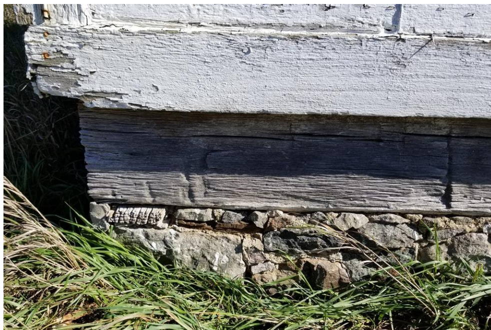
Figure 21: Coursed rubble foundation of the Main Block.
