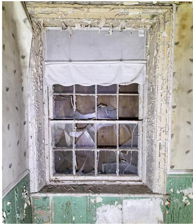
Figure 53: Interior boarded-up window, 12-over-8, with wood panelling below chair rail.
