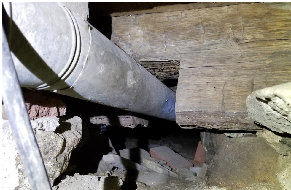
Figure 43: Space below East Wing and beam with adze marks.
