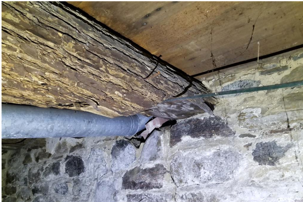
Figure 41: Example of overhead sleeper.
