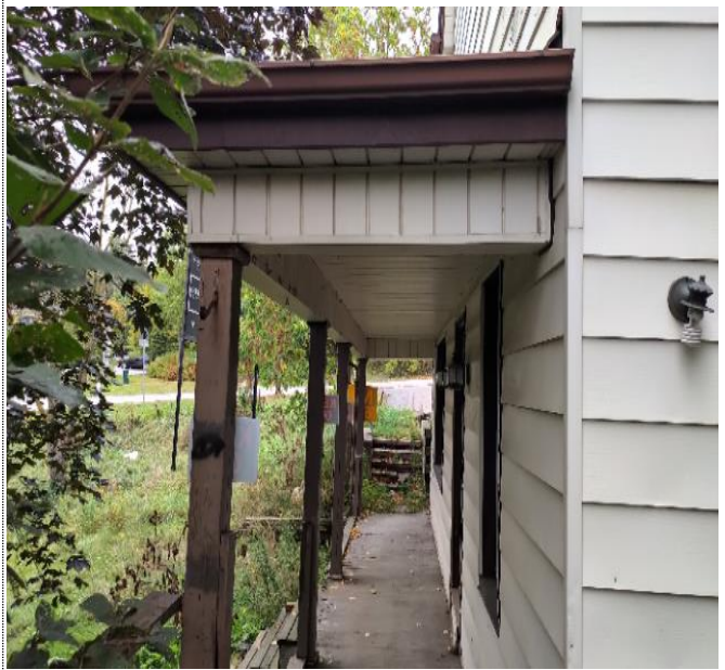
Exterior wood porch concealed with metal siding- South elevation
