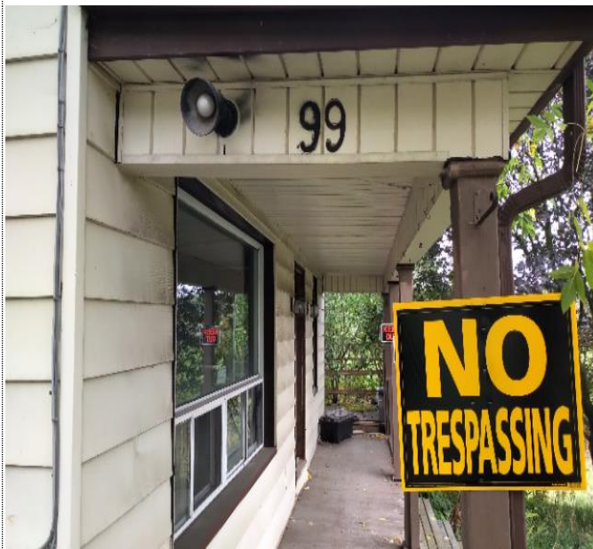
Exterior wood porch concealed with metal siding- North elevation
