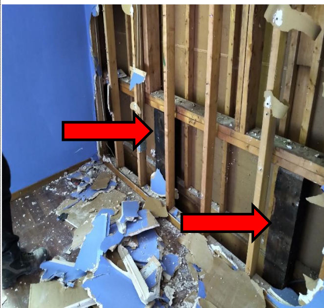
Double wall system forming the newer addition forming the e east elevation. Note, the original timber framing that was found to be extensively charred.
