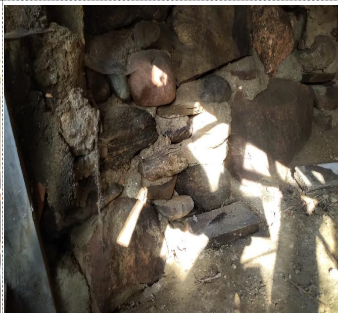
Exterior wood porch supported by loose and deteriorated field stone foundations.
