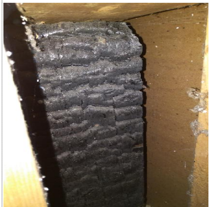
Extensive fire damage to the original exterior wall framing that was partial removed.
