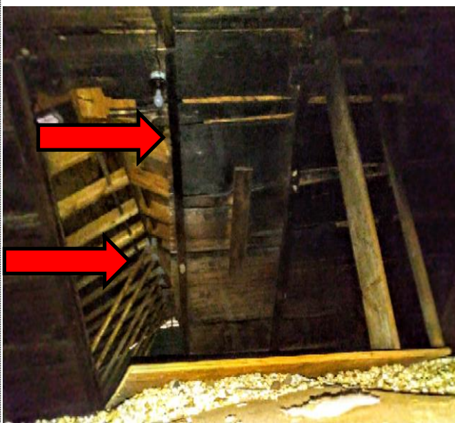
Several wood timber framing and light wood framing have been damaged with fire. It appears that there is visible shrinkage to the timber framing.
