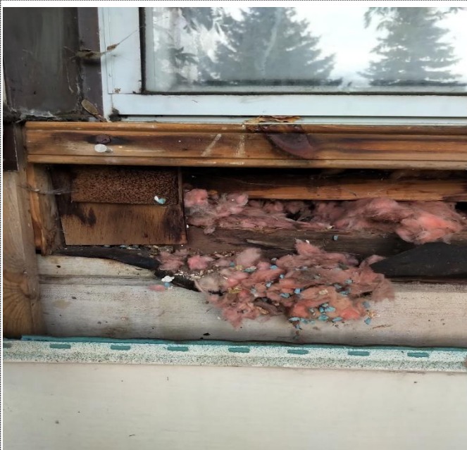
The original sills were removed and replaced. There is water damage and extensive mold growth to the newer lumber and batt insulation. The batt insulation was found to be wet.
