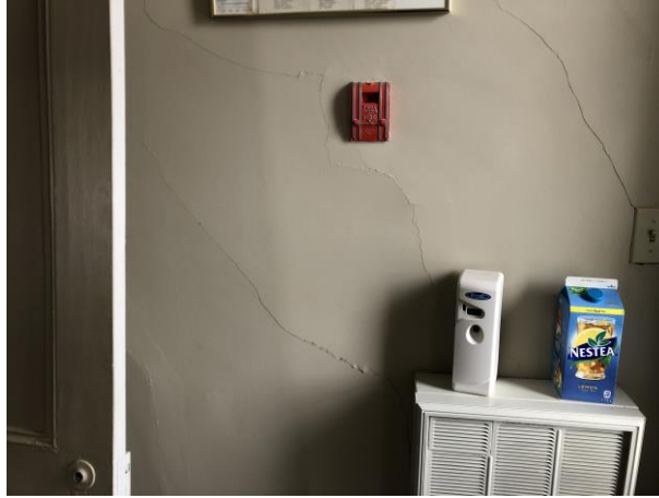
Photo 7- Ground Floor Wall Finish Cracking
