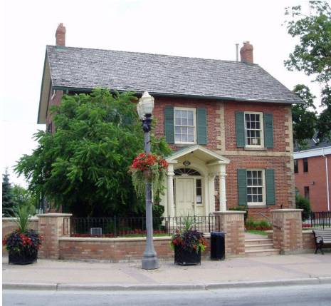
View of the Principal (West) Elevation (City of Vaughan, 2018).
