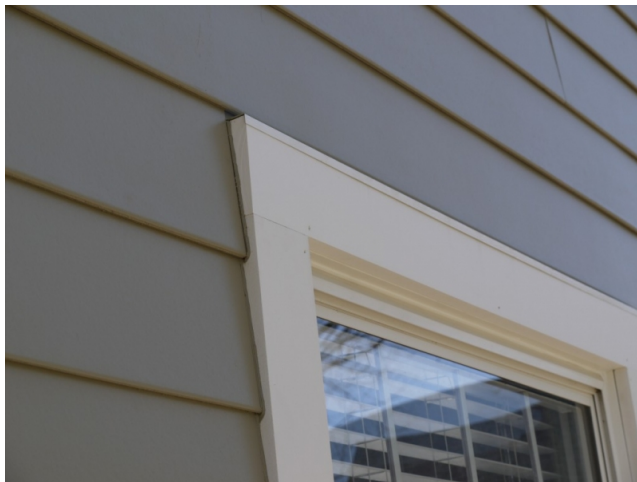
Typical Installation HardiePlank and HardieTrim boards At a window
