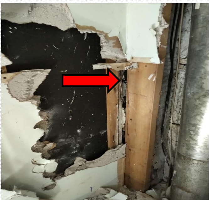
Several alterations have been made to the interior corner connection.
