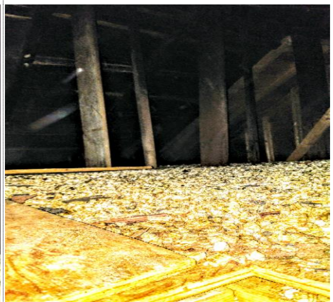
Several wood timber framing and light wood framing have been damaged with fire.
