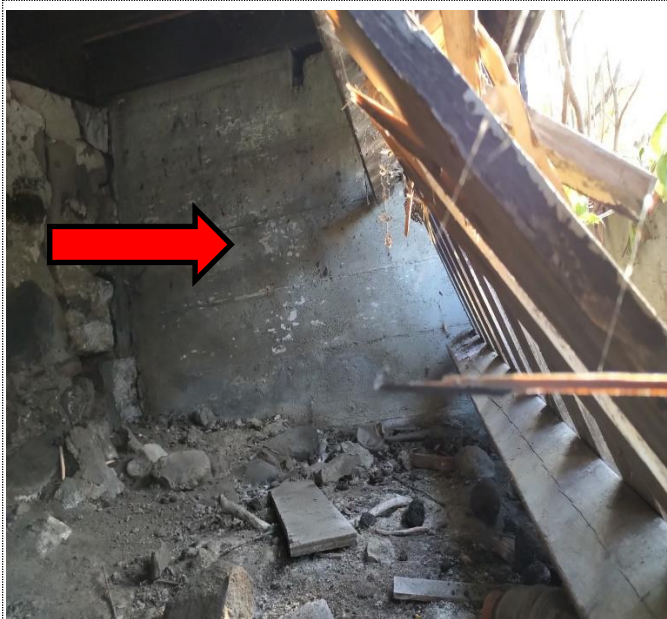
Porch decking supported on cast in place concrete knee wall. Portion of the field stone supporting the porch decking is loose and deteriorated.
