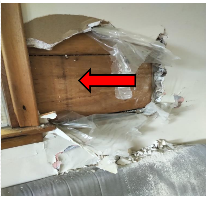
Locally replaced simple plank board forming the exterior walls along the north and west elevations.
