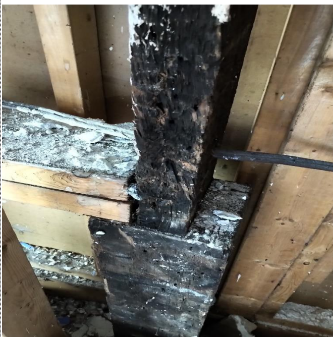
Extensive fire damage and wood rot to the original exterior wall framing that was partial removed.
