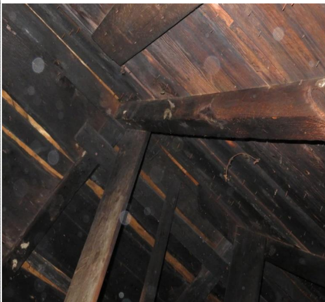
There is extensive fire damage to the original timber rafters and simple plank boards.
