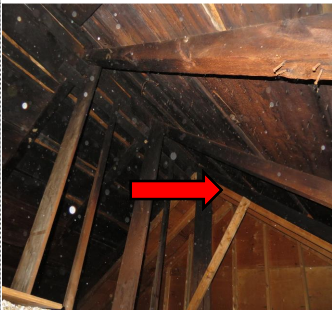
Several wood timber framing and light wood framing have been damaged with fire.
