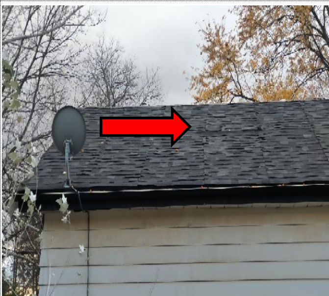
There are obvious sags evident in the roof framing on the north east elevation.
