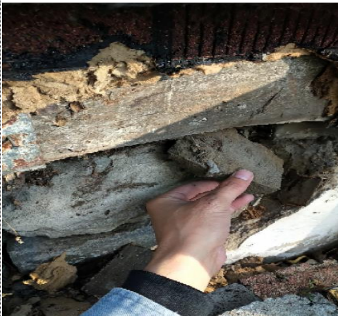
Extensive structural damage to the exposed original field stone. Several stones were found to be loose, as shown.
