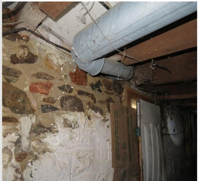
Extensive structural damage to the exposed original field stone. Several stones were found to be concealed and painted with cementitious repair materials, as shown.
