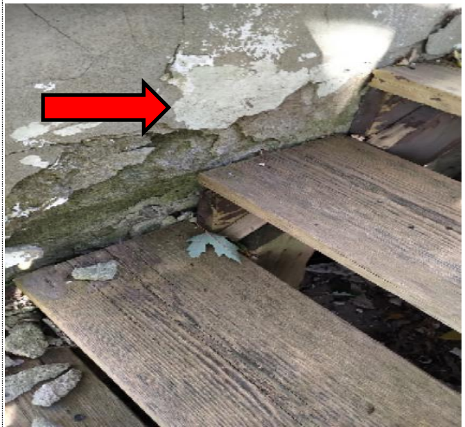
Evidence of spalling and concrete delamination concealing the original loose field stone foundations at the south west corner.
