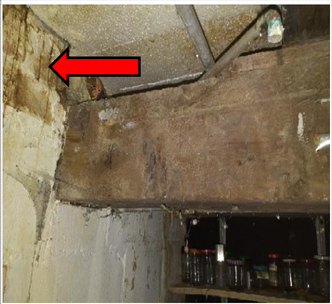
Timber wood beams bearing on block foundation walls below the saltbox addition. Note, evidence of water staining along the upper portion of the foundation walls.
