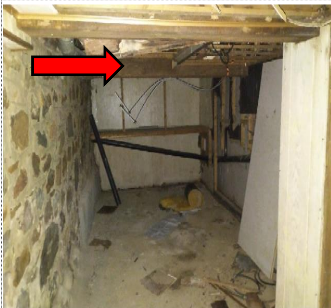
Timber wood beams supporting the wood light framing below the saltbox addition.
