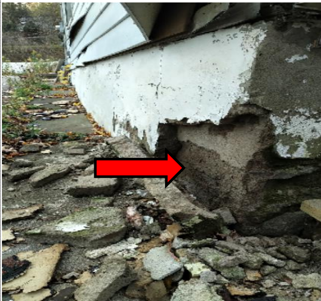
Evidence of extensive concrete deterioration and spalling concrete concealing the original loose field stone foundations. Portions of the foundation walls appear to be bowing outwards.
