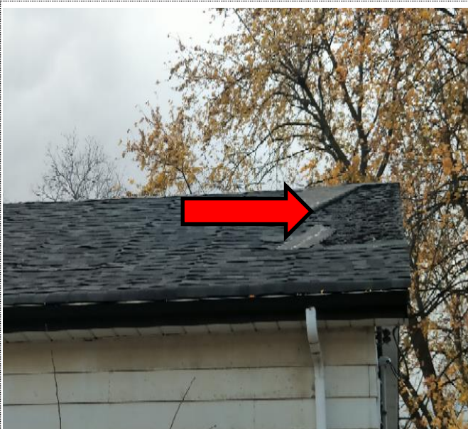
There is an overlay of shingles. The shingles and plywood sheathing where made accessible were found to be deteriorated.
