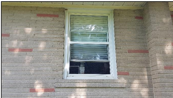
Figure 16: Window on the east elevation with brick sills that are found throughout the house (ASI 2019)
