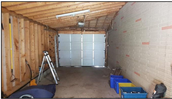
Figure 32: Interior of the garage addition showing the original side wall of the residence (ASI 2019)
