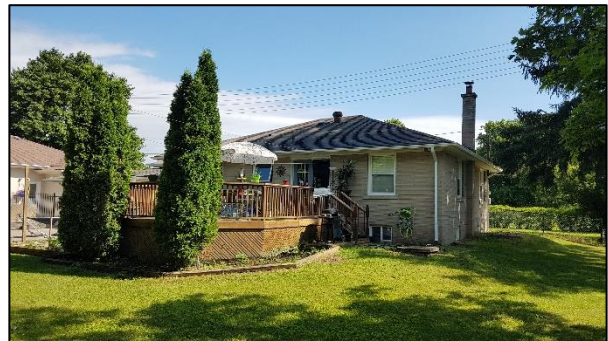
Figure 45: Wooden porch (ASI 2019)
