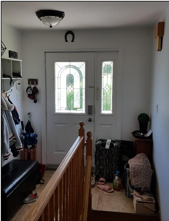
Figure 18: View of the entrance from the south side of the foyer (ASI 2019)
