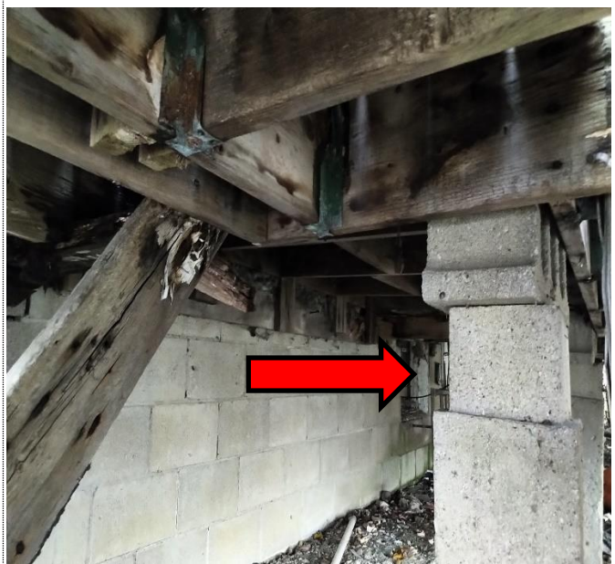
The concrete blocks are temporary supports for the rear addition. The rear addition has settled and is structurally unsafe and in an unsound condition.
