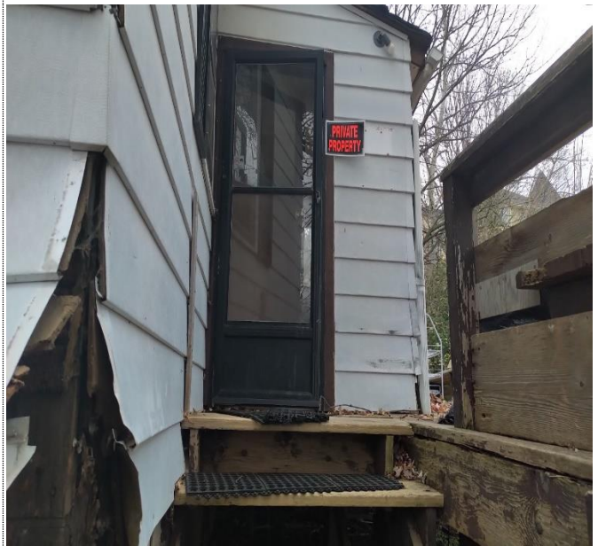
Rear addition bearing on the wood decking and concrete blocks placed above grade.
