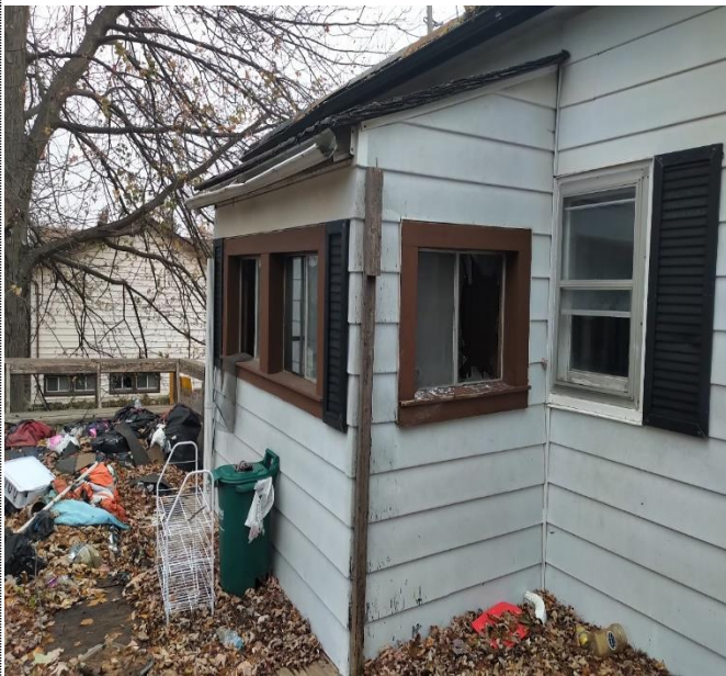
Rear addition, concealed with metal siding and roof assembly concealed with asphalt shingles.
