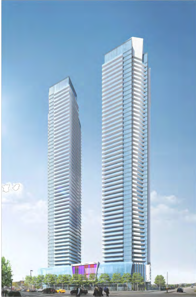
NORTH TOWERS - VIEW FROM NORTHWEST
