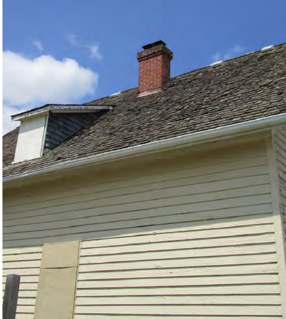
18. South elevation with view of cedar shingled roof and easternmost chimney (ERA, 2019).
