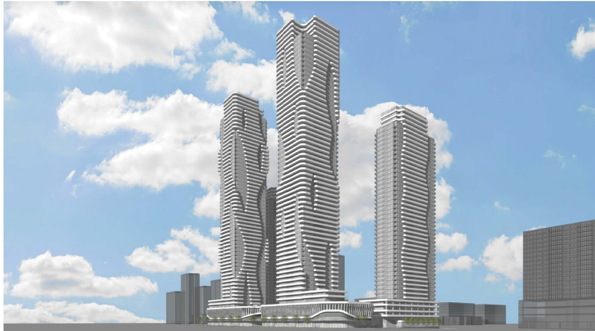
NORTHWEST VIEW FROM REGIONAL ROAD 7
