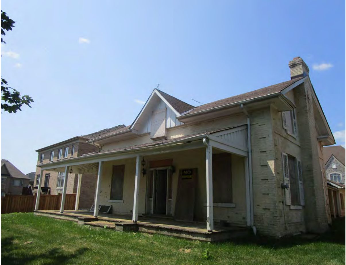
Looking southwest to Bassingthwaite House (ERA, 2019).
