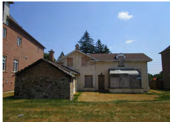
East elevation, including smoke house (ERA, 2019).
