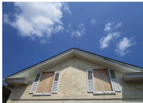
Detail of shutter, sills and soffit on south elevation (ERA, 2019).
