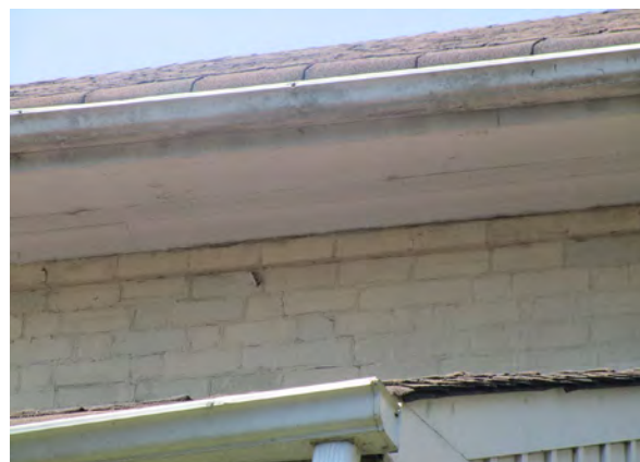
Detail of roof (ERA, 2019).
