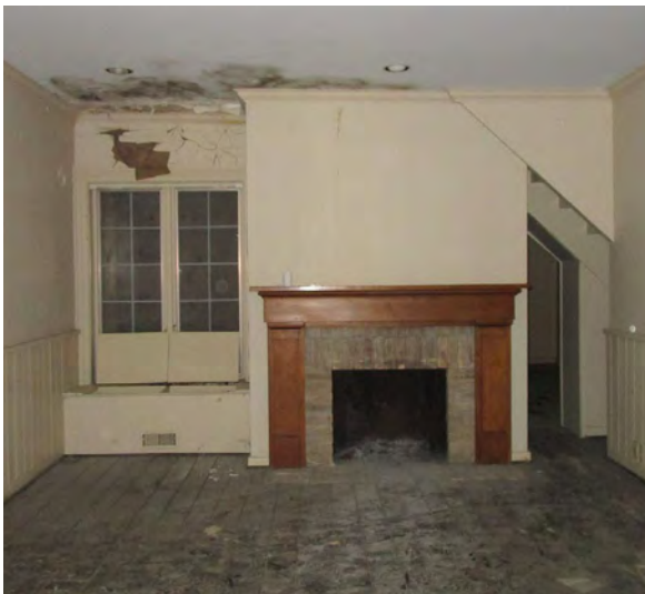
30. View of dining room, with evidence of mould on the ceiling and wall from defective roofing area (ERA, 2019).
