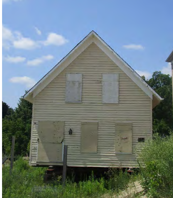
35. George Munshaw House (east elevation) (ERA, 2019).
