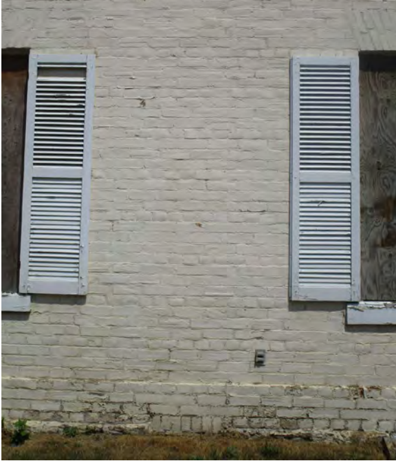
23. North Elevation brickwork and shutters (ERA, 2019).
