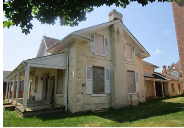
13. Bassingthwaite House - exterior (ERA, 2019).
