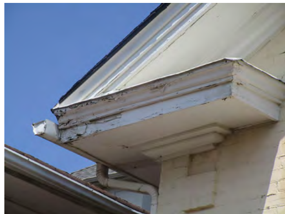
25. Soffiting and moulding on south elevation (ERA, 2019).
