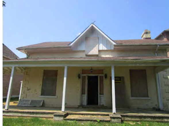
43. Bassingthwaite House main entry along eastern elevation (ERA, 2019).
