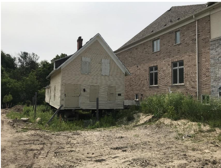
58 Fanning Mills Circle from Western Elevation (Fanning Mills Circle)
