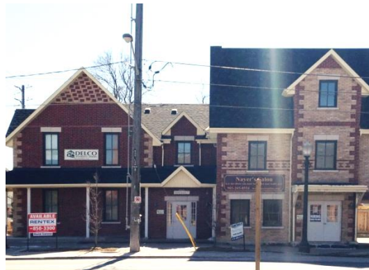
Figure 45 – Reverse Dichromatic Brickwork on the Addition to Historic Structure at 9994 Keele Street , photo taken by AREA, 2015
