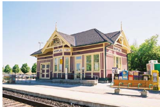
Figure 43 – Decorative Wood Trims at the Historic Maple Station, 30 Station Street , from Maple HCD Vol.1
