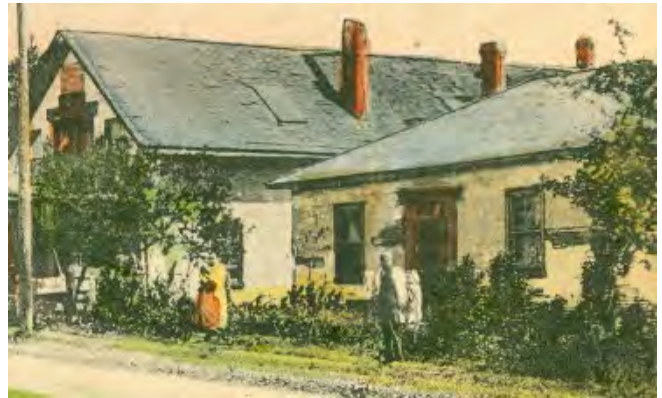
1910 coloured postcard, detail of former Thane Home showing original design features (City of Vaughan Archives)
